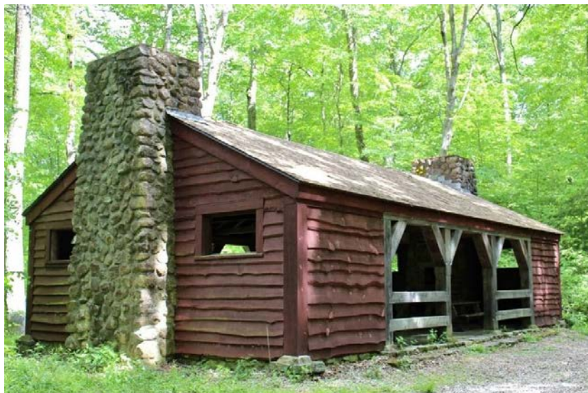
Picnic shelter constructed by DFE and the Appalachian Mountain Club at the backpack campsite. Photo credit: Megan Ruggieri
