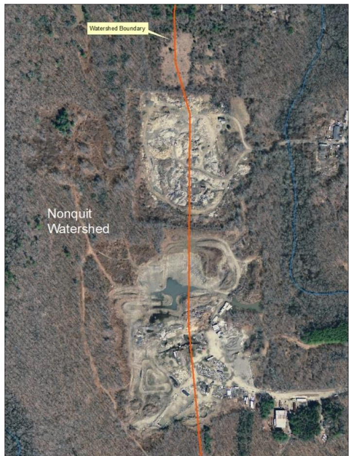
Figure 6: Aerial Image of two Quarries in Vicinity of Nonquit Pond Watershed Boundary
