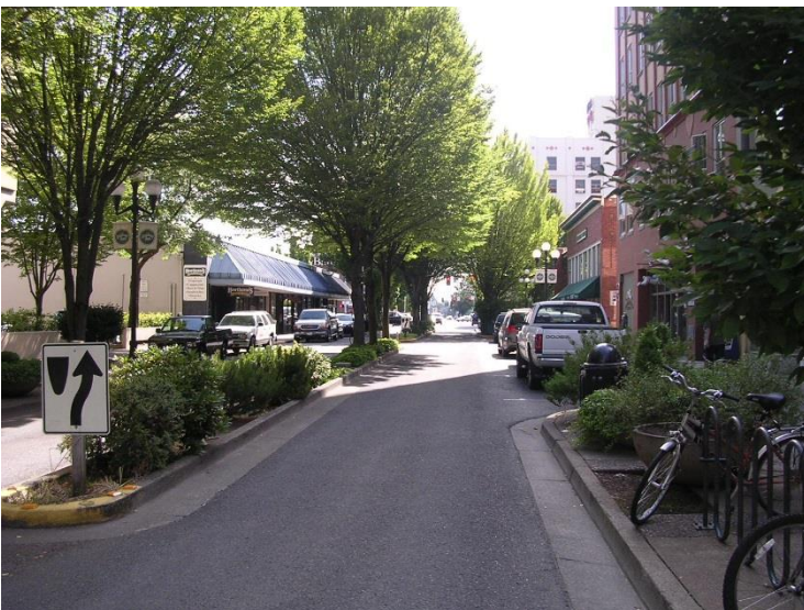
This example of LID shows reduced roadway width and green infrastructure incorporated into the median and sidewalks.
