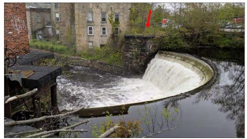
Overview of primary spillway approach and overgrown center embankment (Arrow). – Pare 2019. Centerville Pond Dam (No. 149), West Warwick
