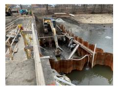
Downstream face of spillway (left) and upstream approach to spillway (right) during repair work at the Canada Pond Dam (No. 093), Providence
