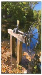
Photo No. 2 Low-Level Outlet Gate Guides and Operator, looking east (upstream), photo taken on September 25, 2019.
