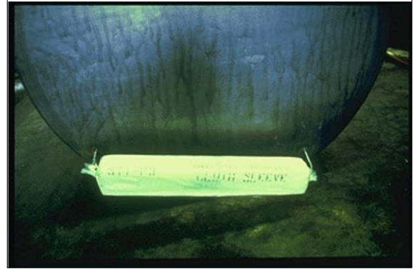
Sample Galvanic (or sacrificial) anode
