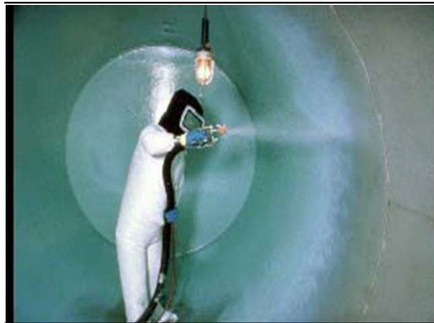
Sample of a Tank being Interior Lined
