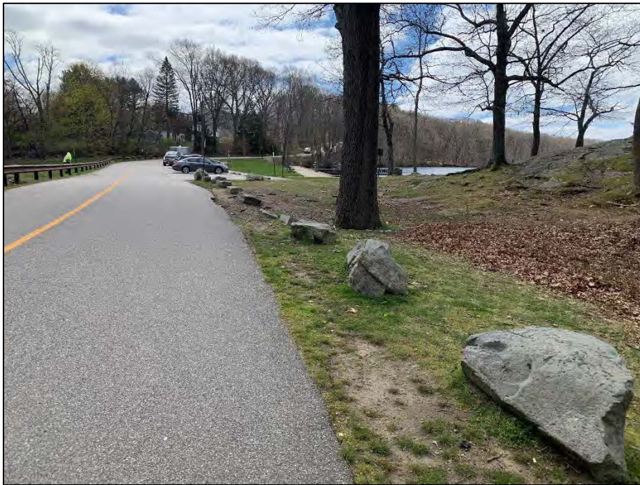
Photo No. 5.: Crest as viewed from the left abutment looking right.
