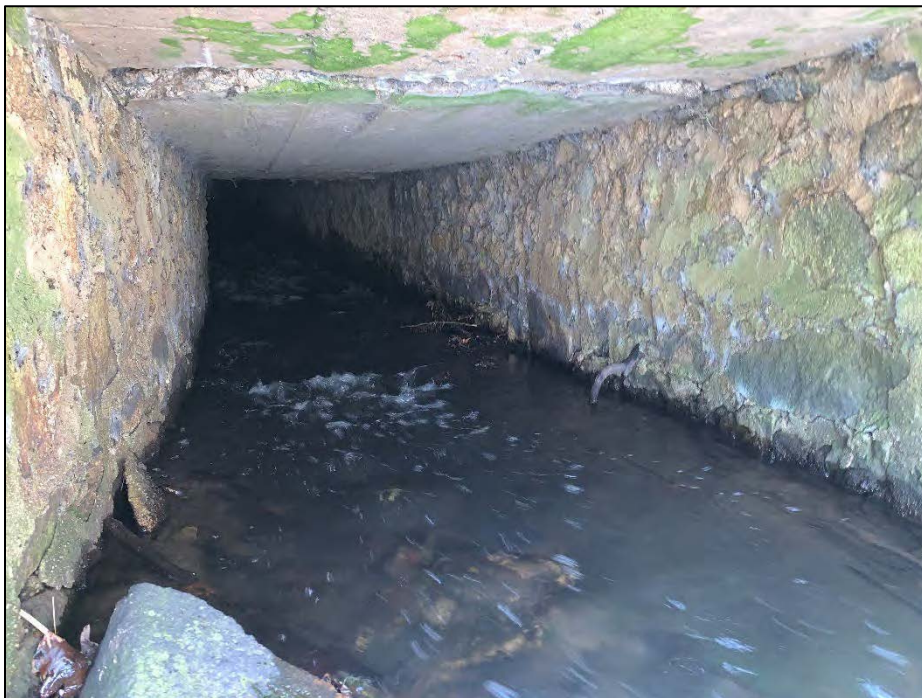
Photo No. 24.: View into primary spillway discharge opening.
