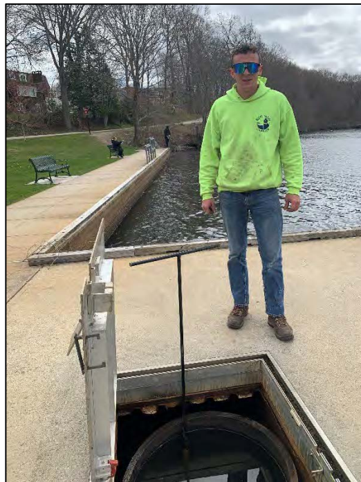
Photo No. 26.: Low level outlet control access hatch.
