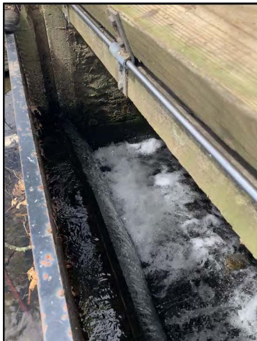
Photo No. 20.: Primary spillway stop log weir section looking left.
