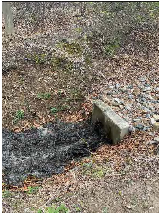
Photo No. 28.: Low level outlet discharge opening following initial gate opening. Note the muddy flow likely from one year of sediment buildup at the intake.
