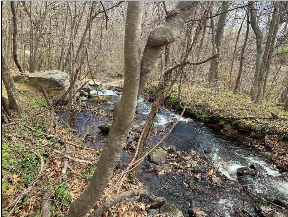
Photo No. 25.: Primary spillway downstream channel looking downstream.
