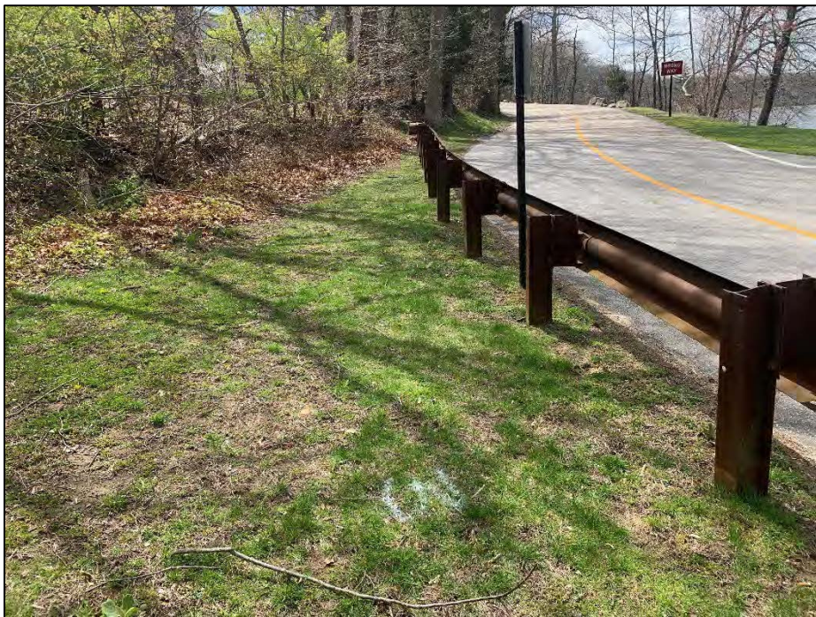
Photo No. 8.: Crest as viewed from the right abutment looking right.
