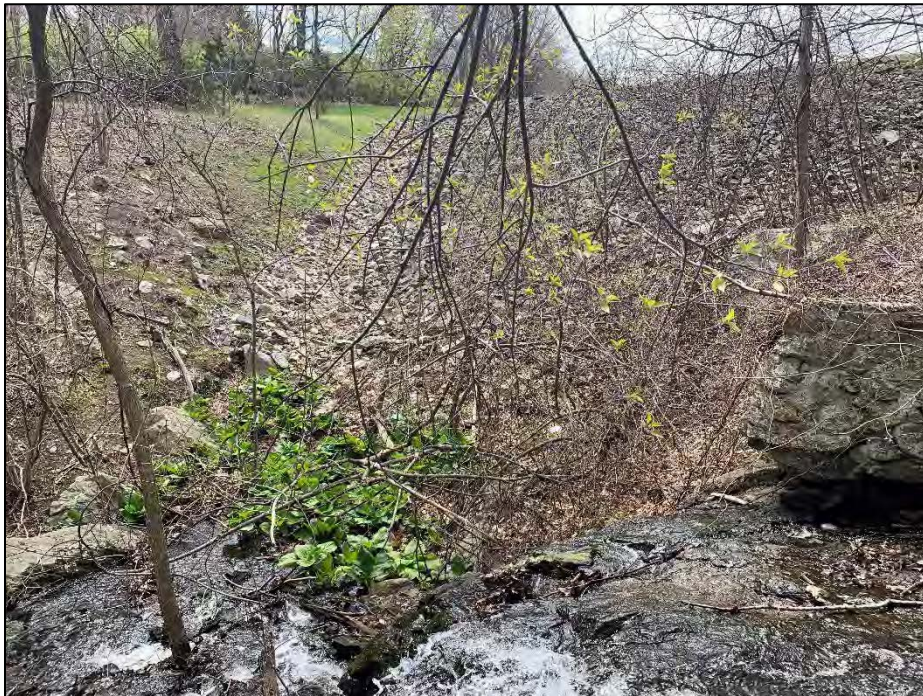
Photo No. 14.: Downstream slope from the primary spillway channel drop off.
