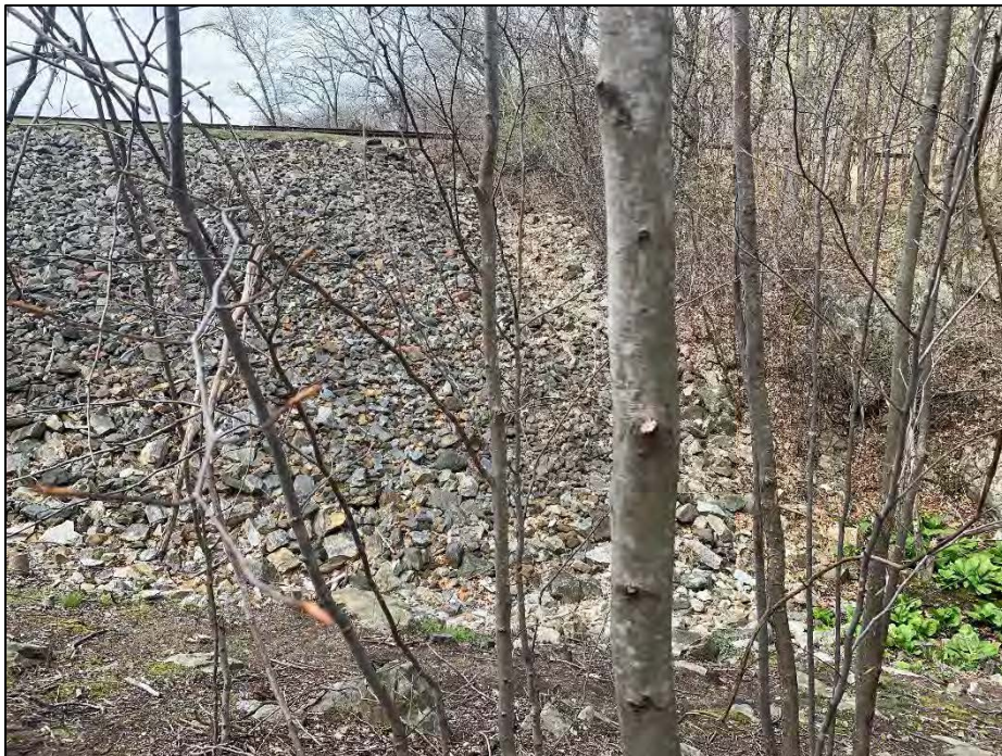
Photo No. 18.: Downstream slope as viewed from beyond the right groin looking upstream and slightly left. Note the wetland vegetatoin along the toe.
