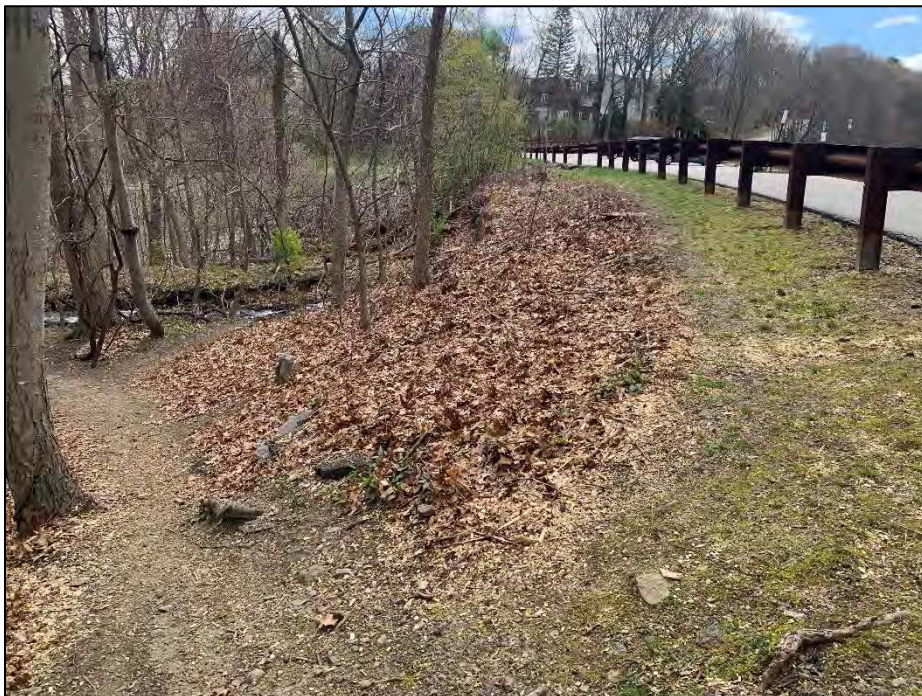
Photo No. 12.: Downstream slope from the left abutment looking right. Note the deadfall cover and tree growth.
