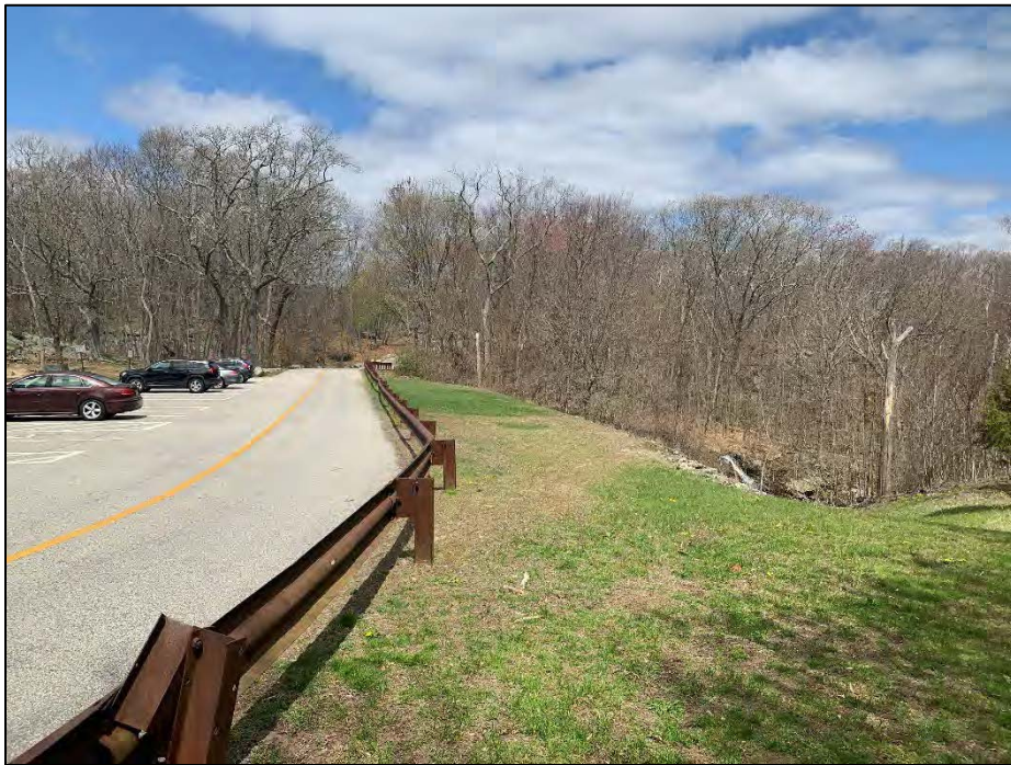
Photo No. 11.: Crest as viewed from the right abutment looking left.
