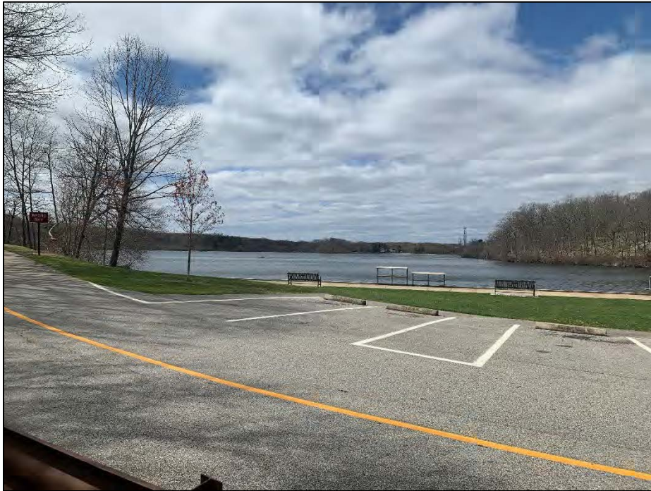
Photo No. 9.: Crest and impoundment as viewed from the right abutment looking upstream.
