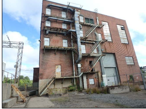
Photo 2 Overview of the south side of the Control House on September 9, 2018, as viewed from the south.
