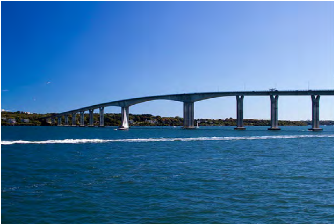
Jamestown Bridge West Passage
