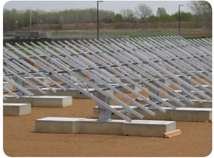
Figure 5: High-density Pre-cast Concrete System (photo: Solar FlexRack)
