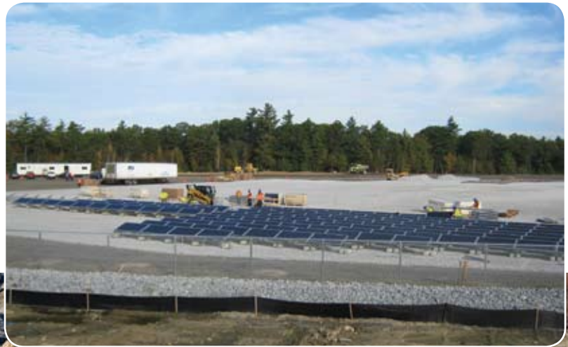
Cathartes Private Investments: Construction of 4.5-MW Solar PV Array (photo: Nexamp)
