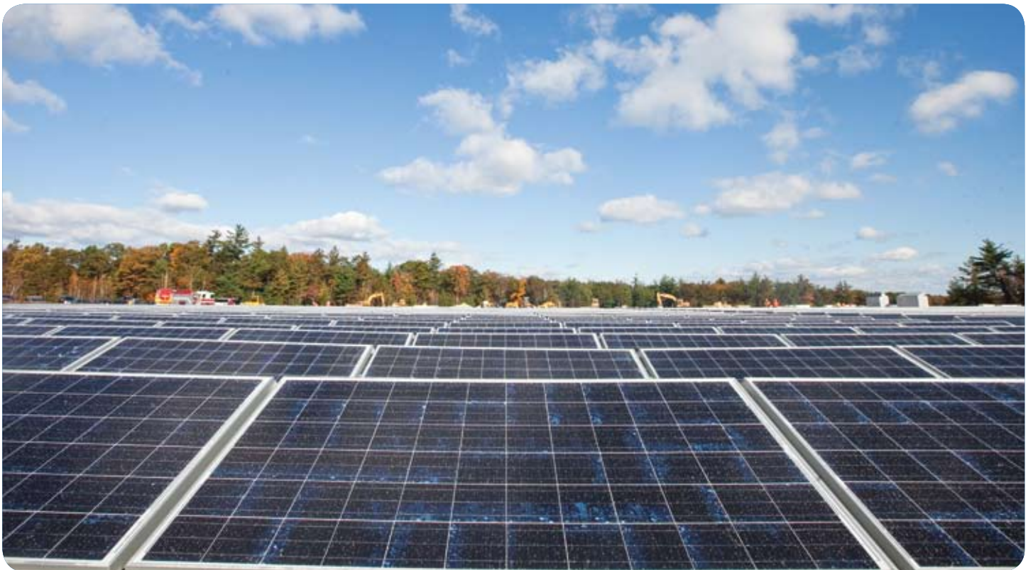
Cathartes Private Investments: 4.5-MW Solar PV Array (photo: Tara Morris Images)
