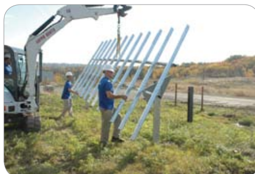
Figure 6: Driven Pile Mounting Structure (photo: Solar FlexRack)
