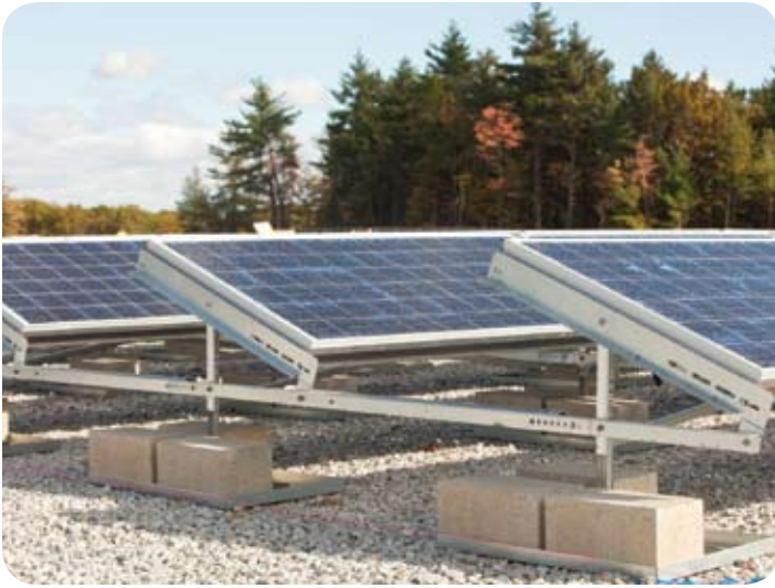
Figure 4: Massachusetts-manufactured Panel Claw Mounting System (photo: Nexamp)
