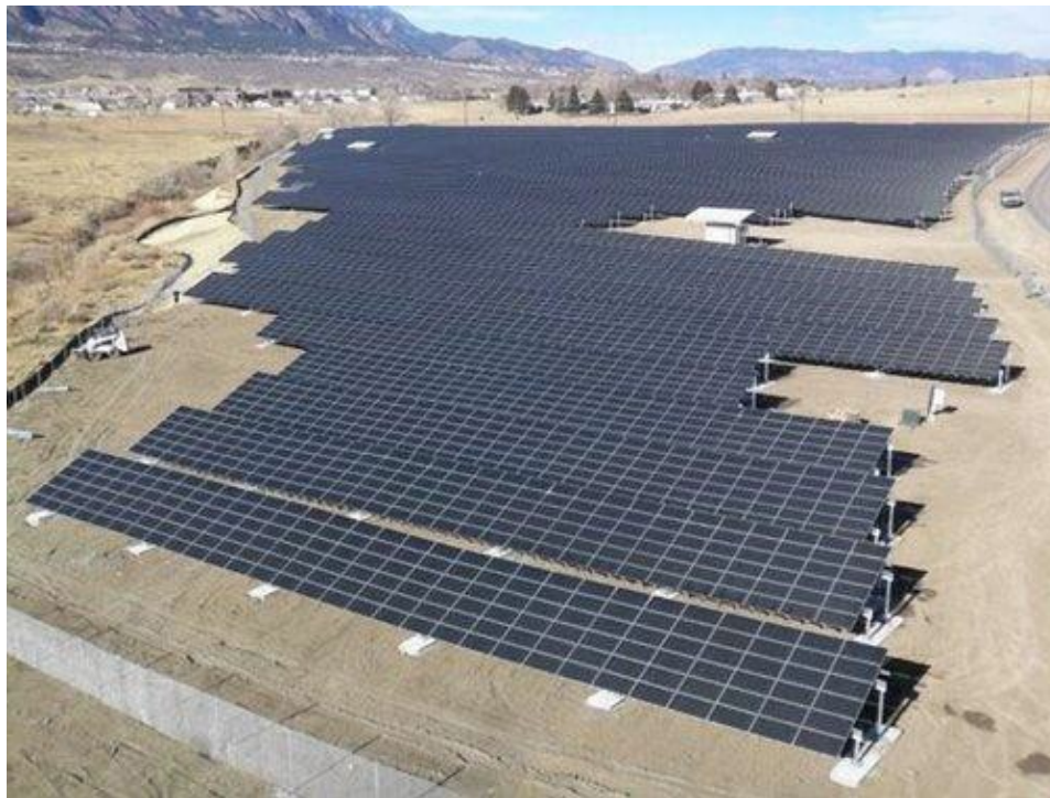
Figure 3-6: 2-Megawatt peak (MWp) PV system with fixed tilt on former landfill in Fort Carson, Colorado.
