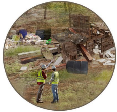
ASSESSING CURRENT SITE/SOIL CONDITIONS
