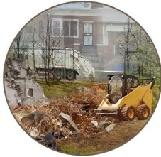
CLEANING SITE - REMOVAL/RECYCLING DEBRIS
