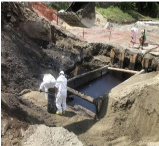
Image 7. Oily soil excavation efforts.
