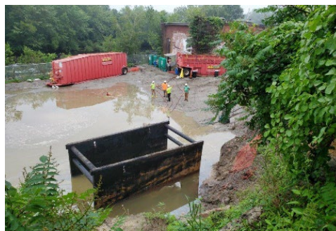
Image 8. Flooded excavation site.
