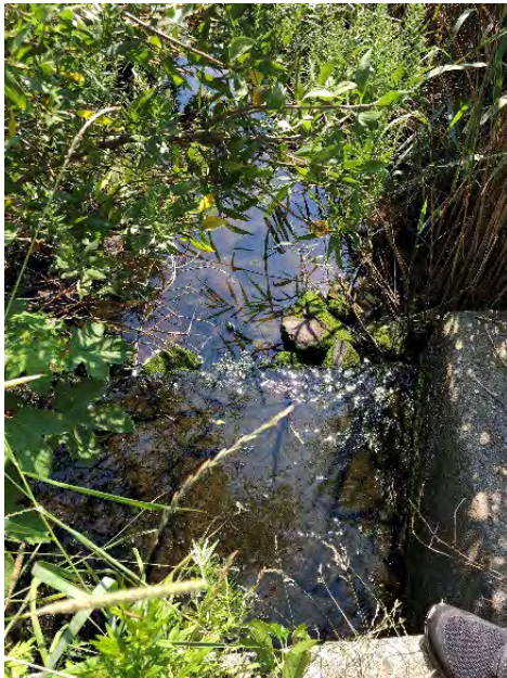
Figure 5: Source 5-008, drainpipes at the extension of Parker Avenue in Warren RI.
