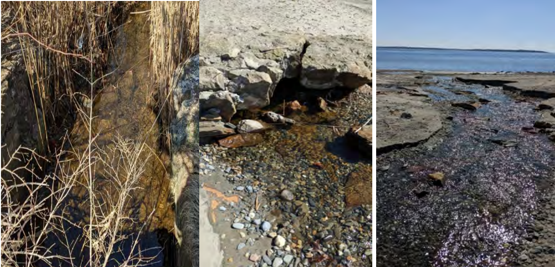
Figure 6: Source 1-017, a culvert fed by outflow of an upland pond at the south end of Rocky Point Beach.
