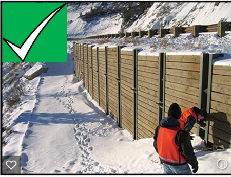
* Well engineered retaining wall.
