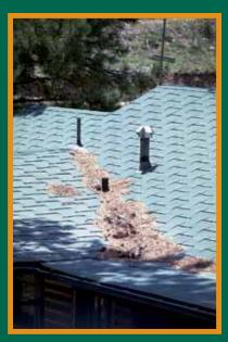
Figure 14: Clearing pine needles and other debris from the roof and gutters is an easy task that should be done at least once a year.
