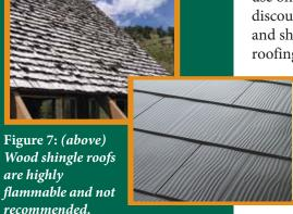
Figure 8: (above right) Class A roofing materials including tile, clay, concrete, slate and asphalt shingles are fire-resistant options. Photo: CSFS
