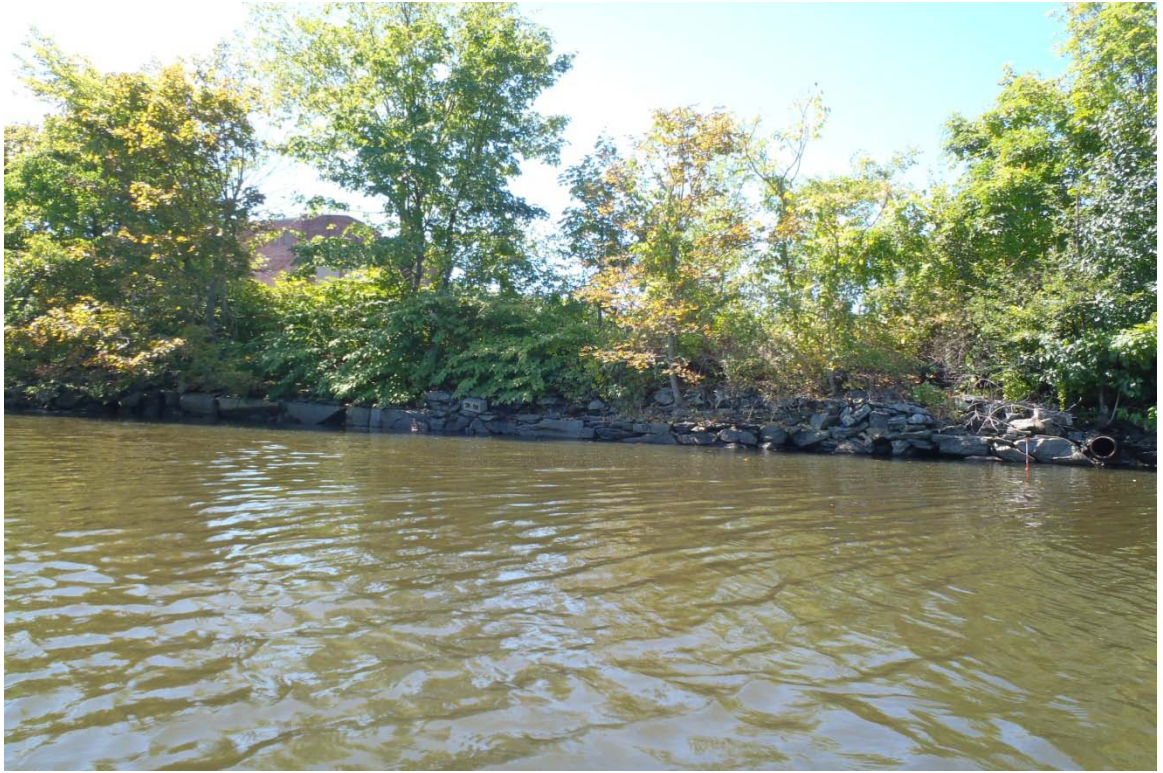
Photo 1: Shoreline area along FGPA where intermittent sheen is observed.
