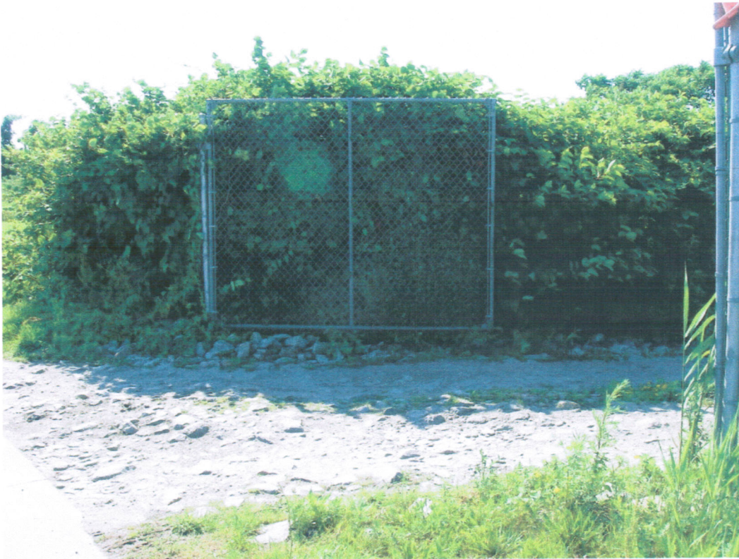
Photo 1 – Entrance off Park Avenue
