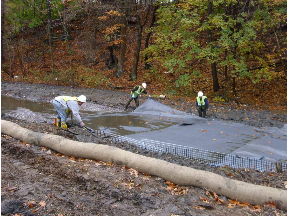
Photograph No. 7 Installation of geotextile over geogrid in the sluiceway (11/5/10).
