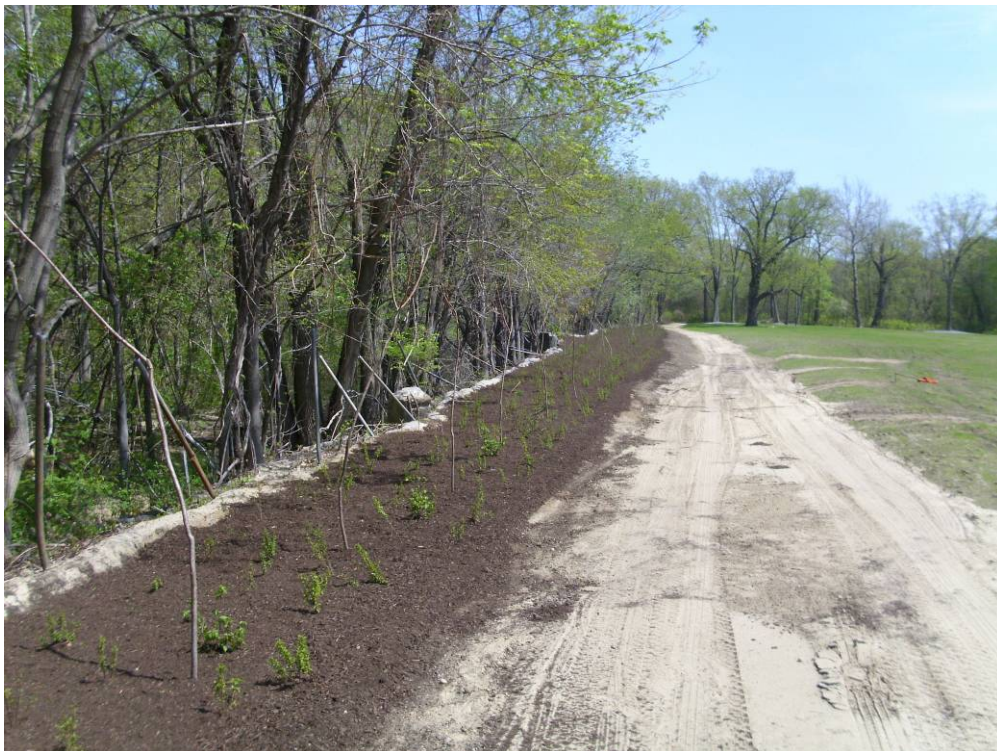
Photograph No. 30 Mulched landscaping along the proposed bike path (5/6/11).
