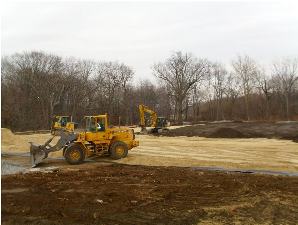
Photograph No. 22 Installation of loam and fill material (11/23/10).
