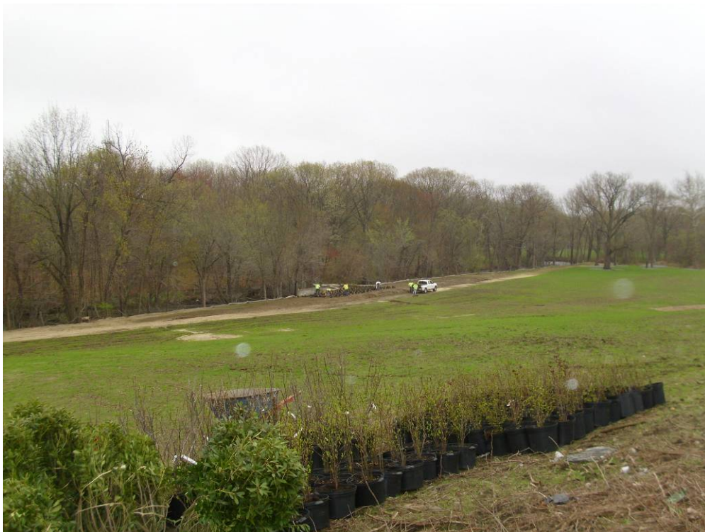
Photograph No. 26 Landscaping the site (4/28/11).
