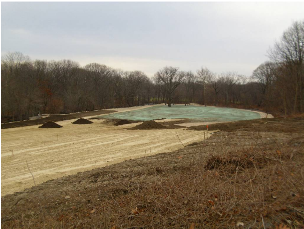
Photograph No. 24 Hydroseeded eastern portion of the site (12/3/10).
