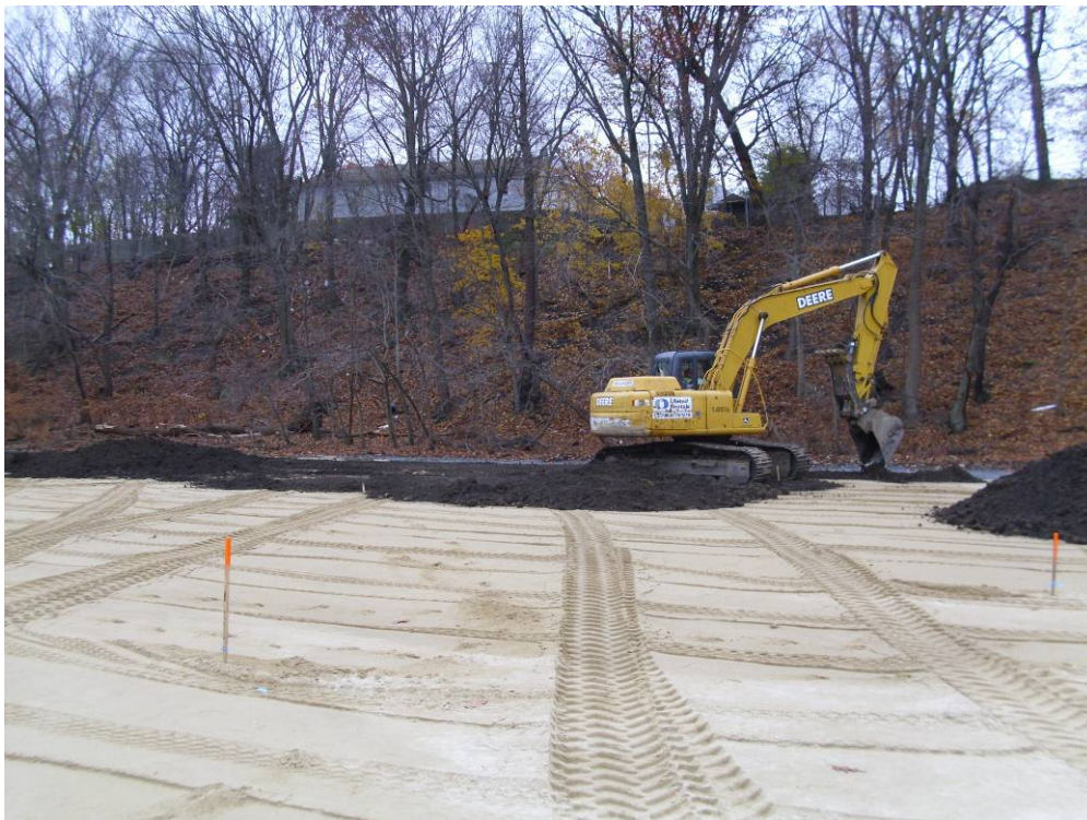
Photograph No. 20 Installation of loam over fill material (11/22/10).
