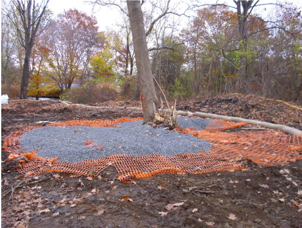
Photograph No. 13 Engineered barrier around mature trees left in place (11/10/10).
