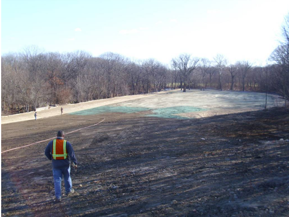
Photograph No. 25 Hydroseeding the central portion of the site (12/8/10).
