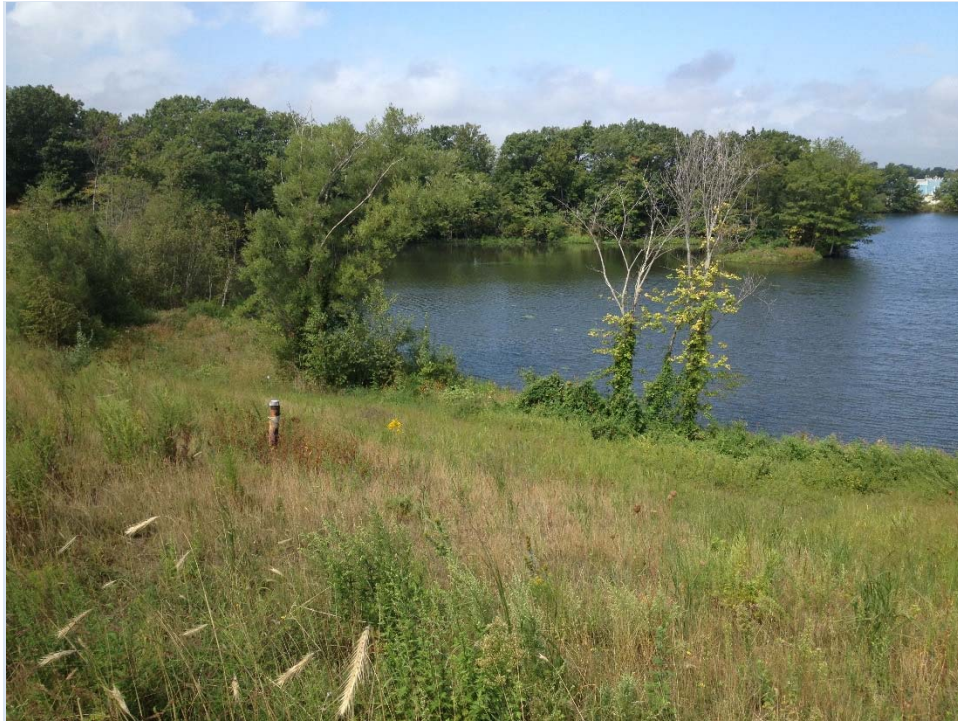
1. Restored fringe wetlands and Phase I cap, view to northwest.
