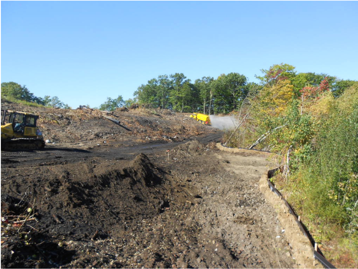
0940. Water truck applying dust control at Areas 3 and 4, looking south
