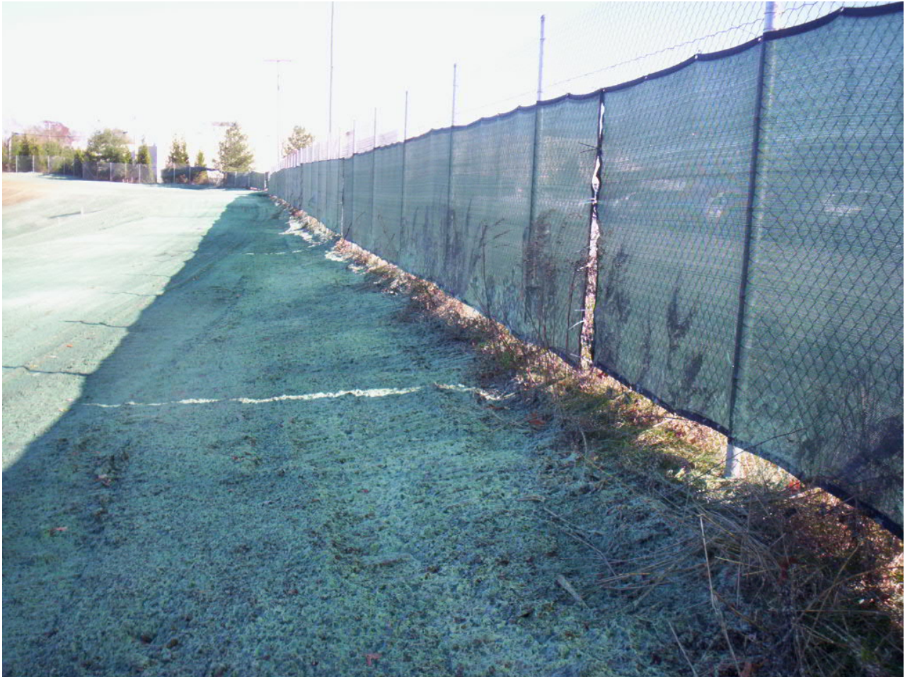
1675. Hydroseeding along the outside of the high school fence, looking east
