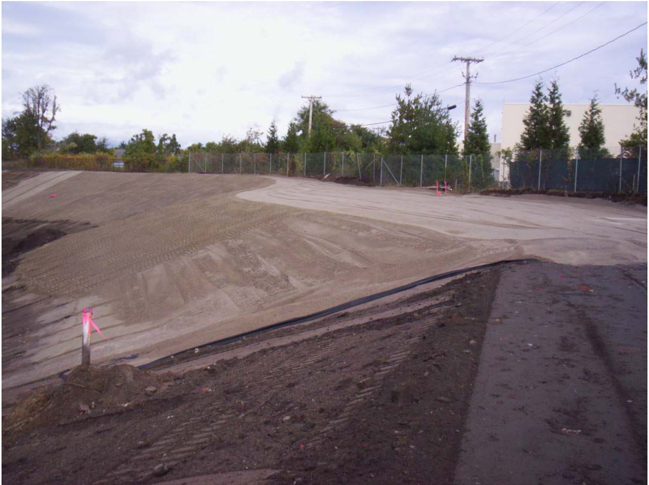
1048. Cover soil placement completed on upland cap of Area 5, looking northeast
