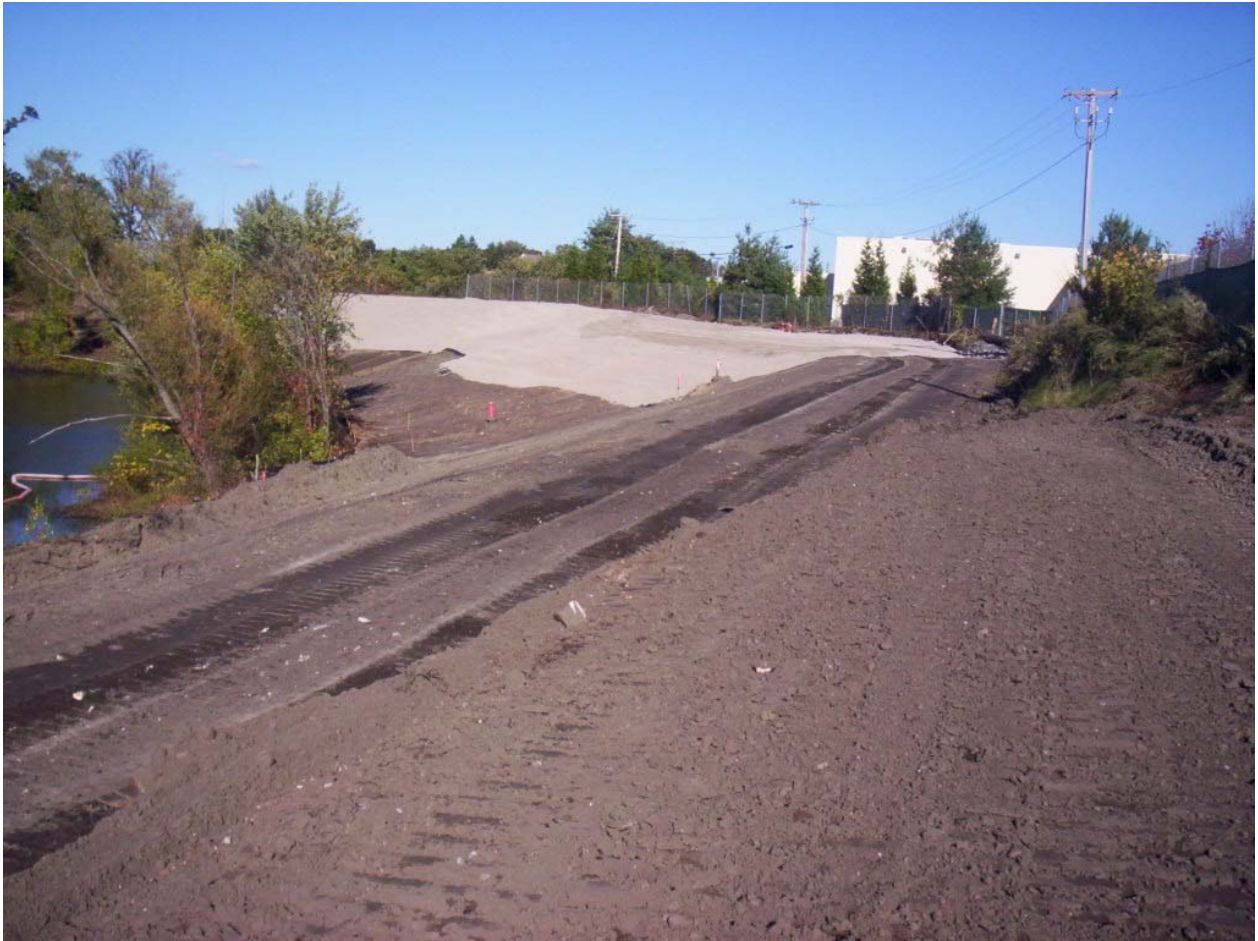
1039. 2 nd lift of cover soil placed on upland cap of Area 5, looking northeast
