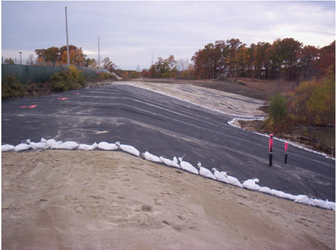
1597. Looking southwest at the installed geomembrane at Area 4
