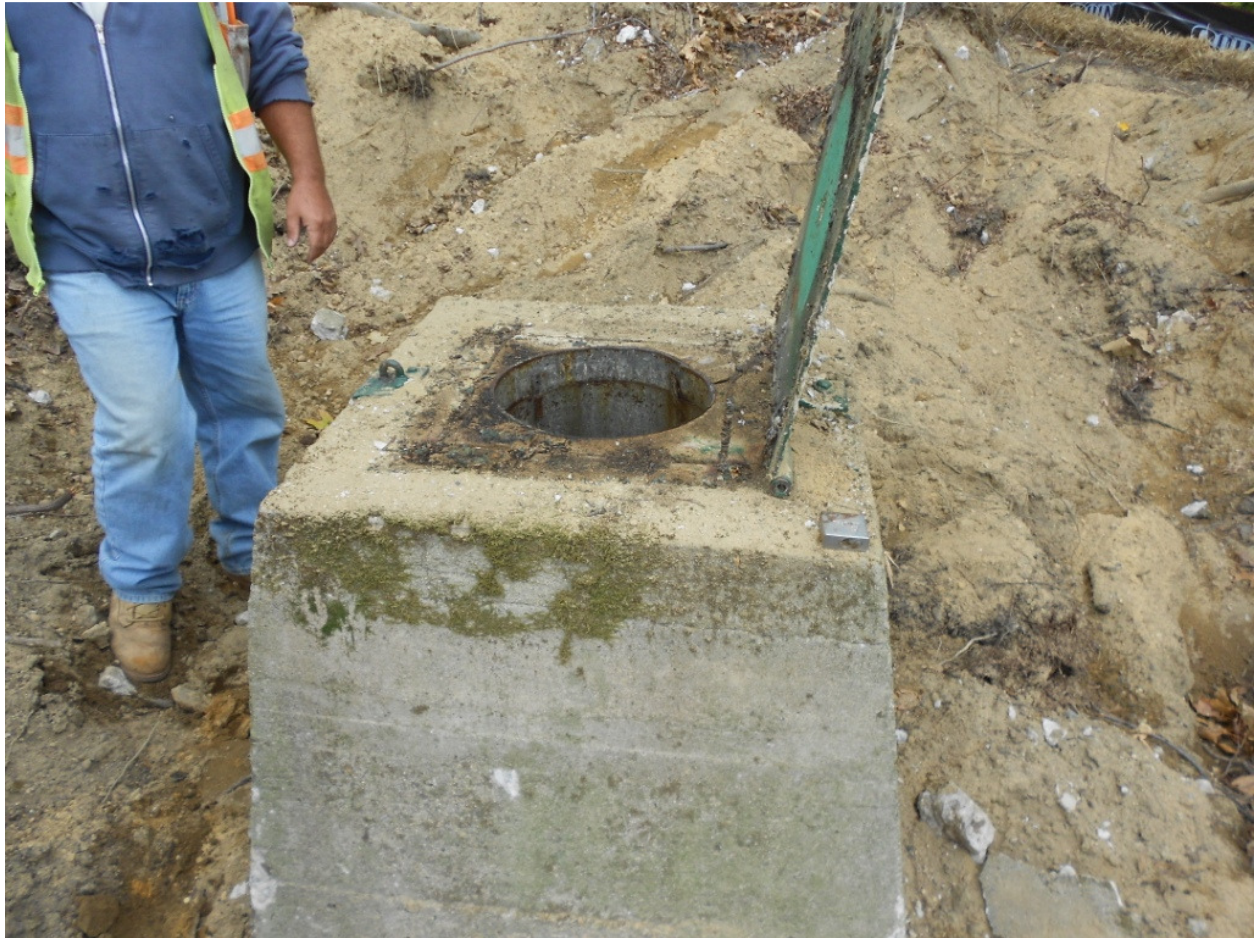
0918. Concrete vault containing well at the beginning of the peninsula
