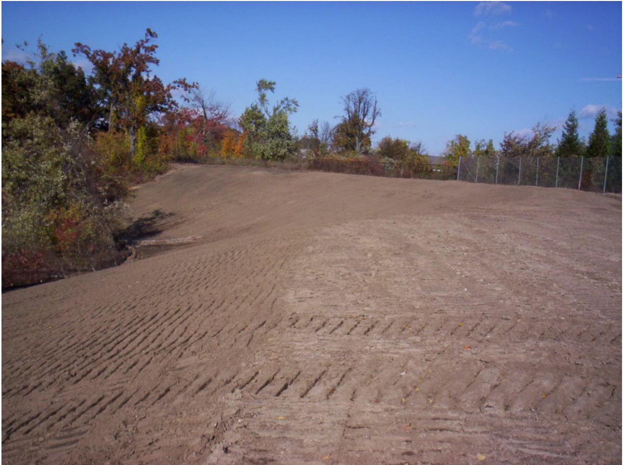
1574. Looking north at repaired topsoil on Area 5
