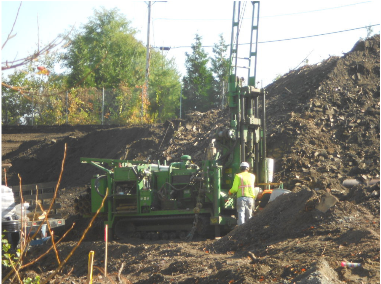
1018. Subcontractor Geosearch set-up to install new well MW-243S, looking east
