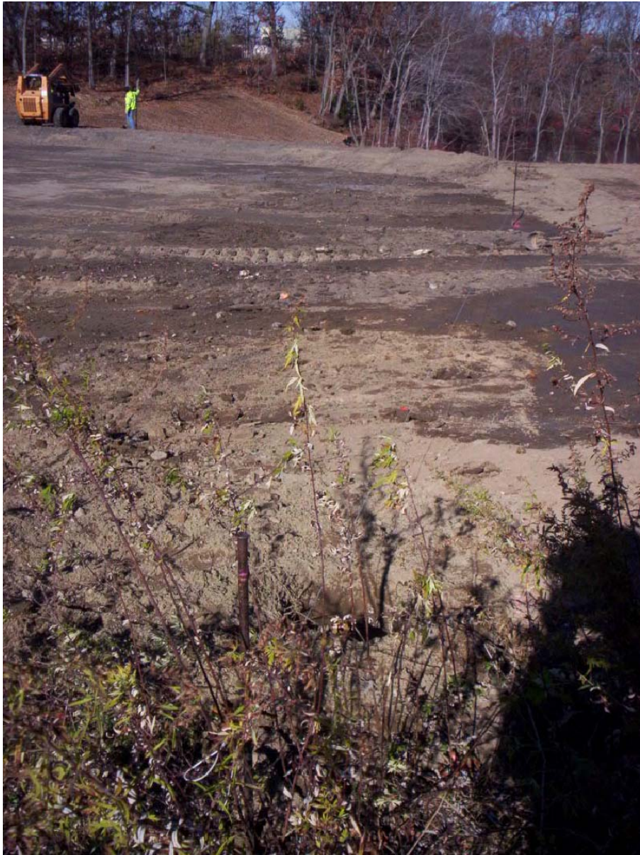
1661. Costco staking out and augering fence post holes, looking northwest
