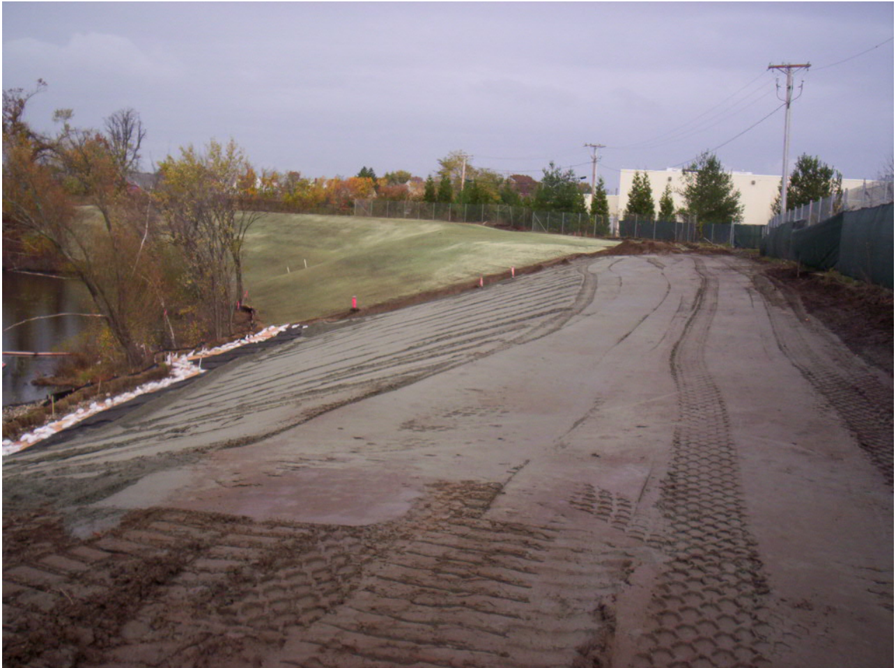
1626. Protective soil graded and compacted at Area 4, looking northeast
