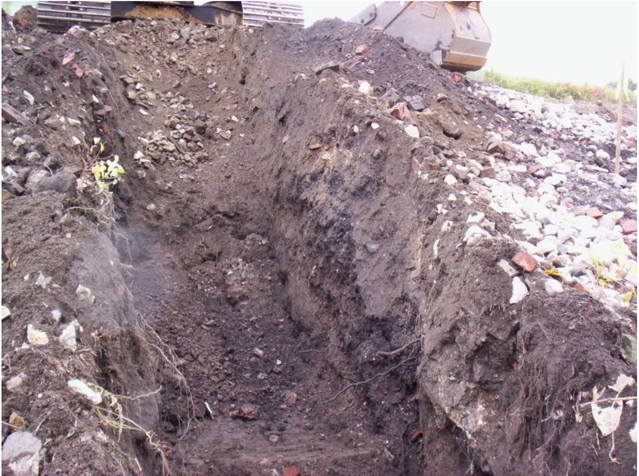
1514. TP 9, excavated 4 ft bgs
