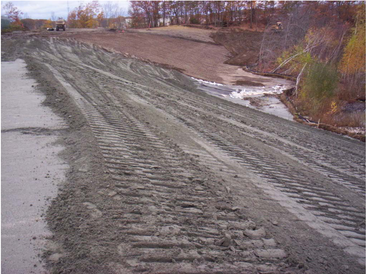
1632. Eroded slopes repaired at Area 4 protective soil, looking west
