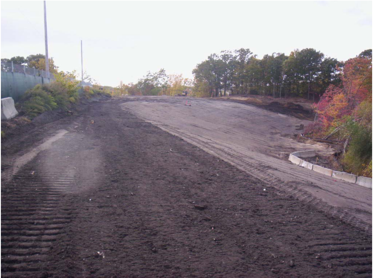
1057. Looking southwest at sub-grade preparation at Area 3 and Area 4
