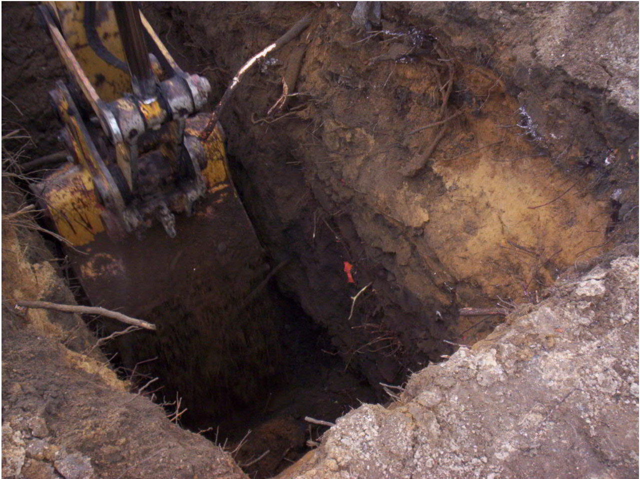
1526. TP 5, excavated 5 ft bgs
