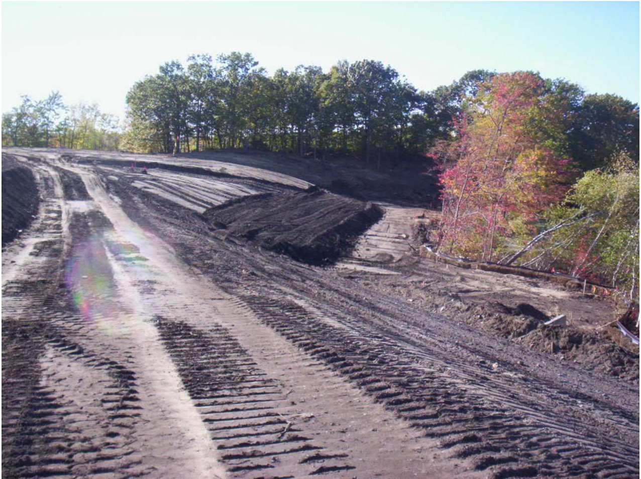
1040. Looking southwest at sub-grading at Areas 3 and 4
