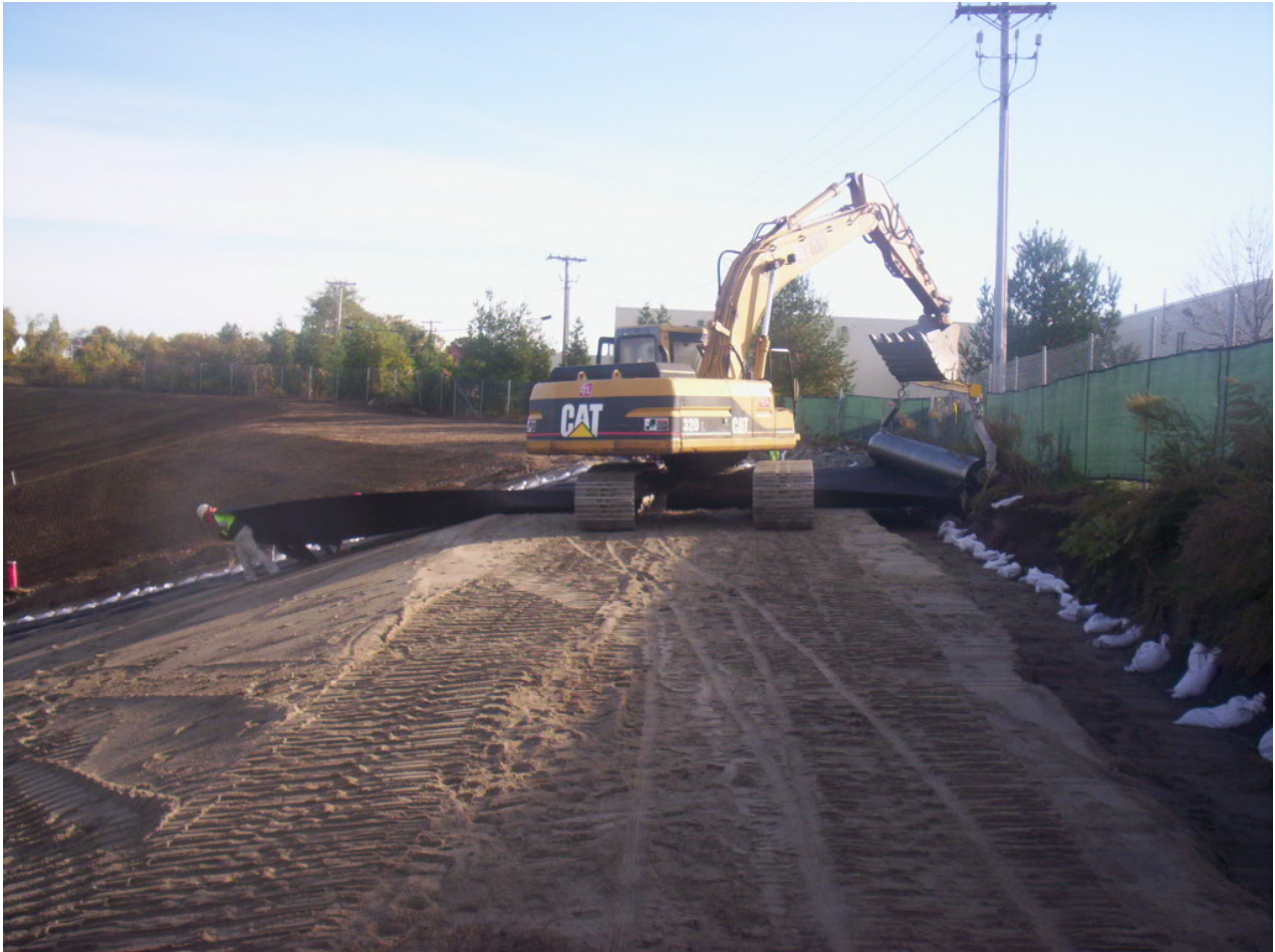
1578. Begin installing geomembrane at Area 4, looking east
