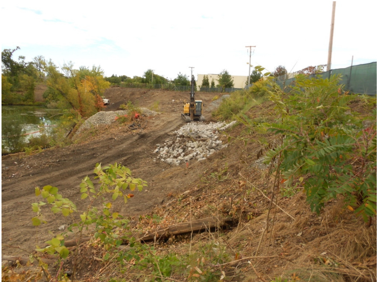
0915. Excavator breaking up concrete pieces with hoe ram attachment, looking northeast
