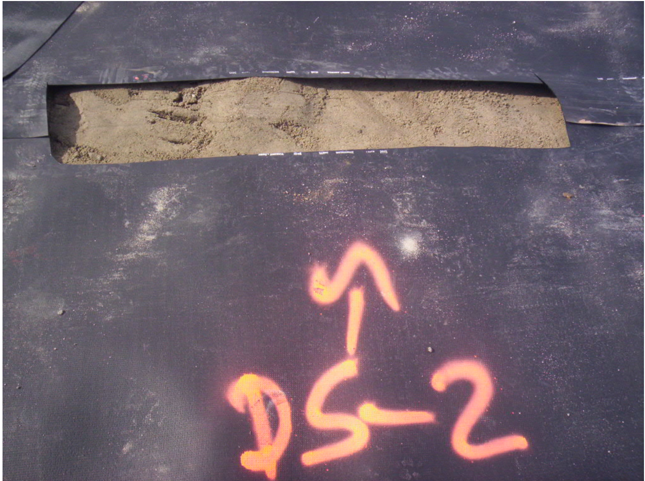
1591. Location of destructive test (DS-2)
