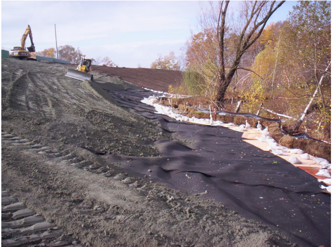
1619. Placing and grading protective soil at Area 4, looking southwest
