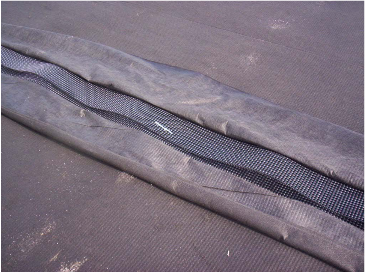
1609. Plastic ties used to tie adjacent panels of drainage geocomposite
