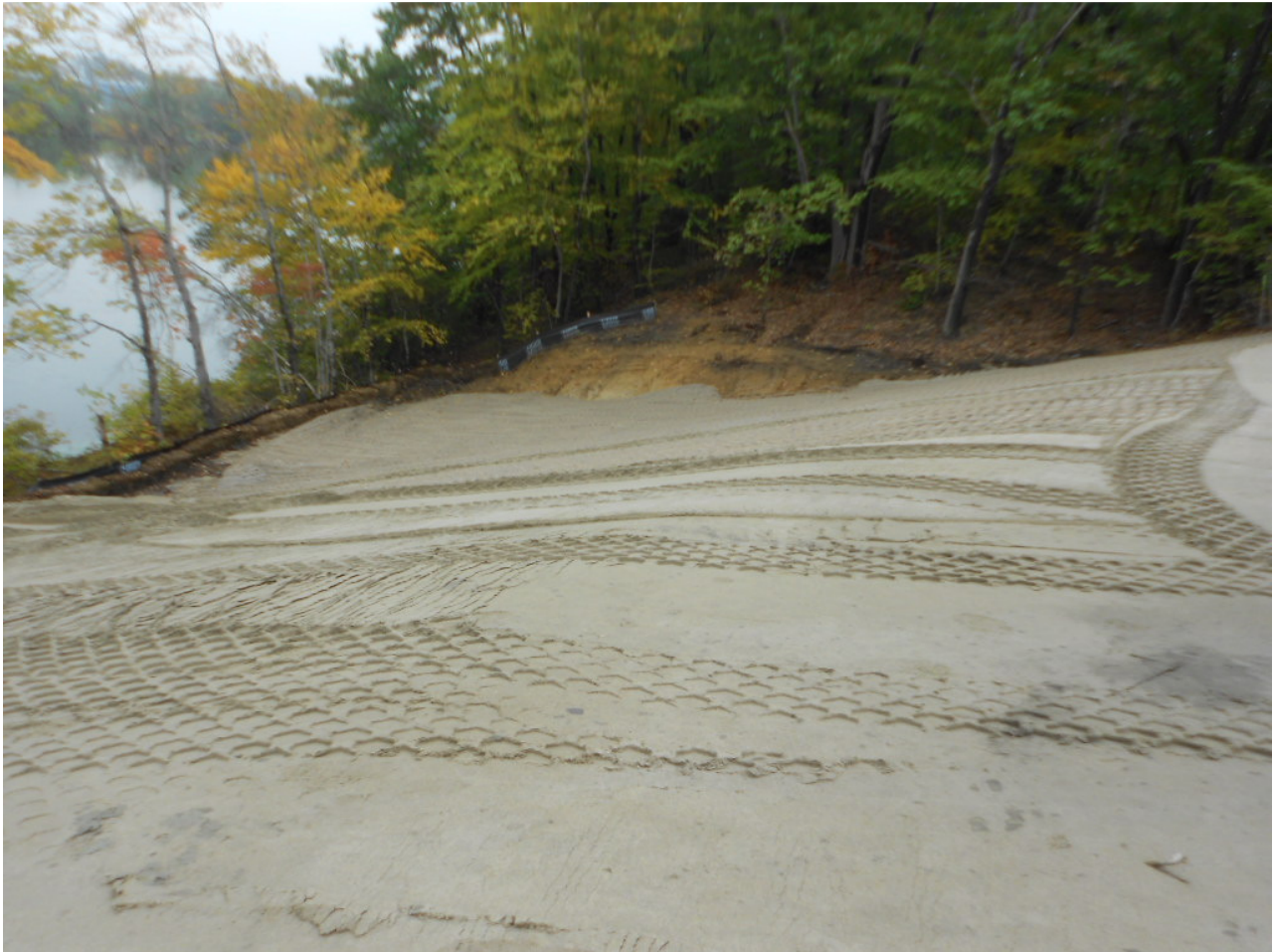
0996. Area 2 cover soil compacted, looking northwest
