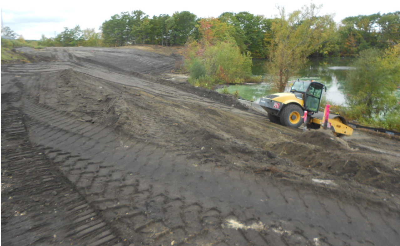
1030. Roller compacting sub-grade at Area 4, looking southwest
