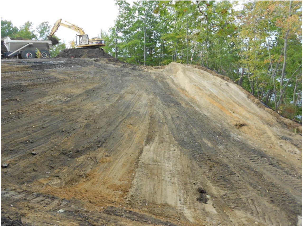
0959. Loading out soil from Area 2, looking south
