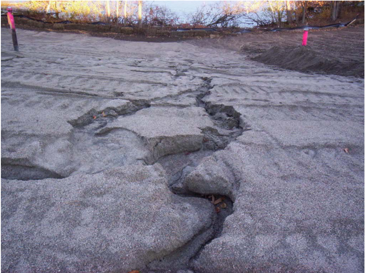
1568. Buffer sand erosion at Area 4 from the rain event during the weekend of 10/20/12 and 10/21/12, looking north
