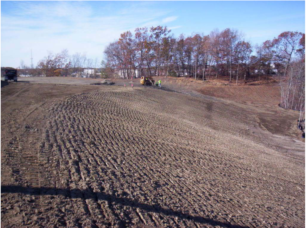
1660. Costo augering fence post holes, looking southwest
