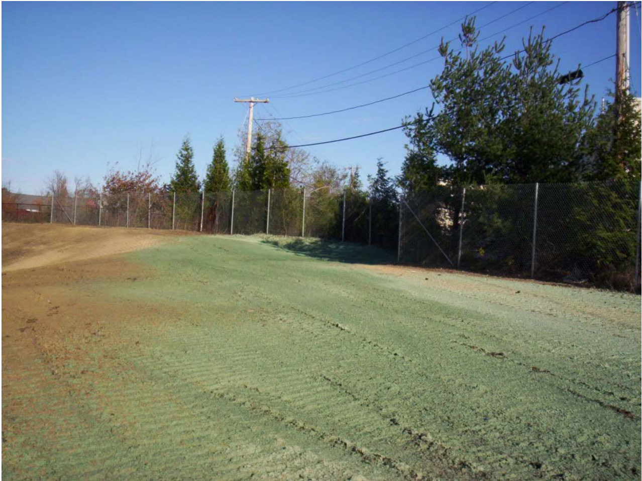
1684. Area hydroseeded near the fence at Area 5, looking east
