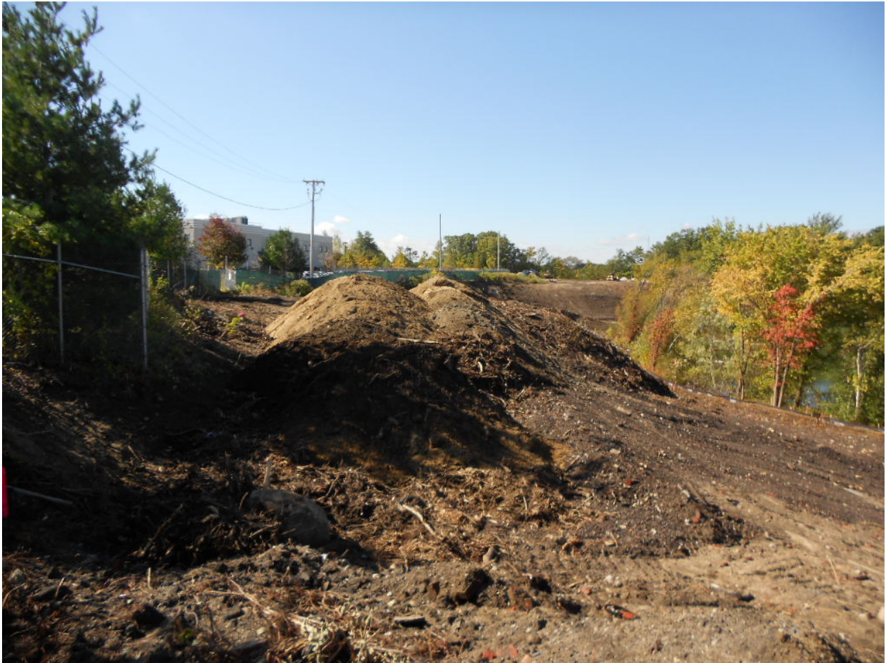
0970. Excavated soil from Area 2 stockpiled at Area 5, looking southwest
