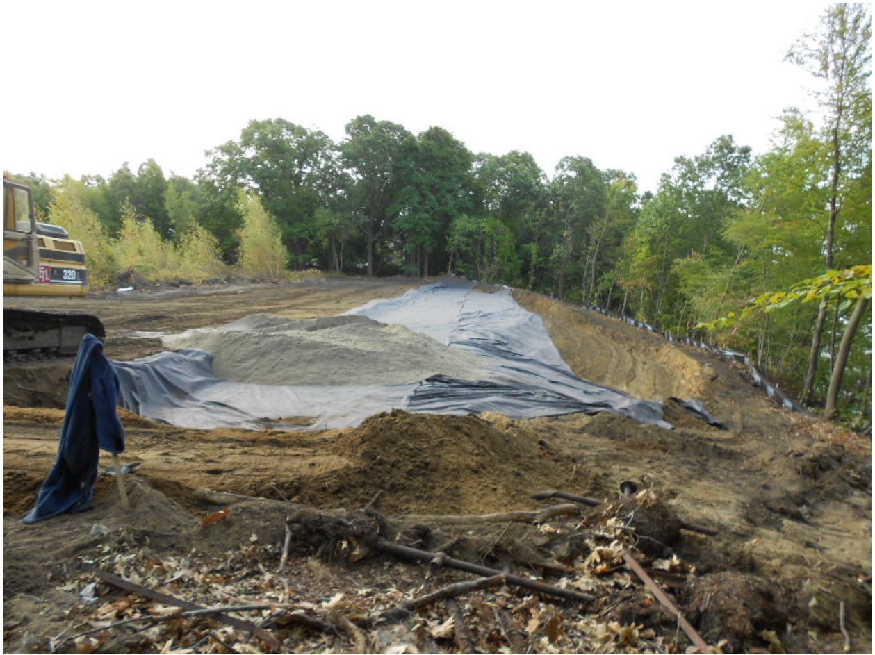
0947. Cover soil and geotextile installed at Area 1, looking south
