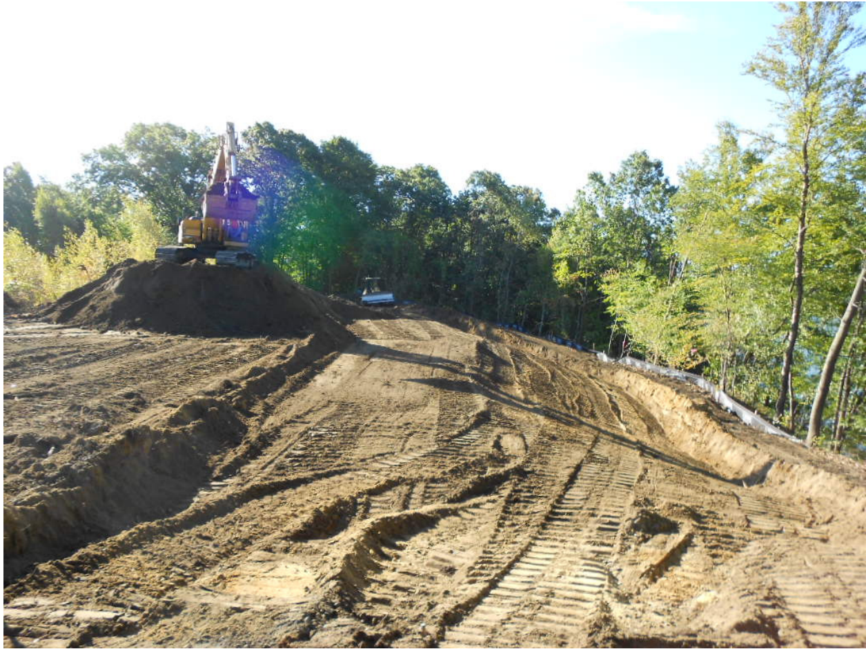
0934. Looking south at the Area 1 excavation
