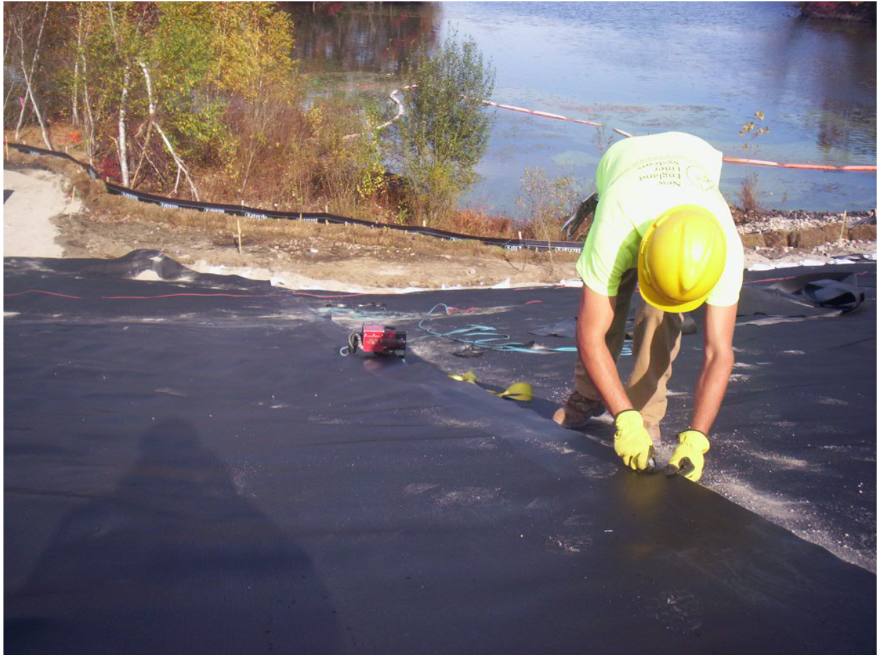
1583. Fusion welding end seams during geomembrane installation at Area 4, looking north
