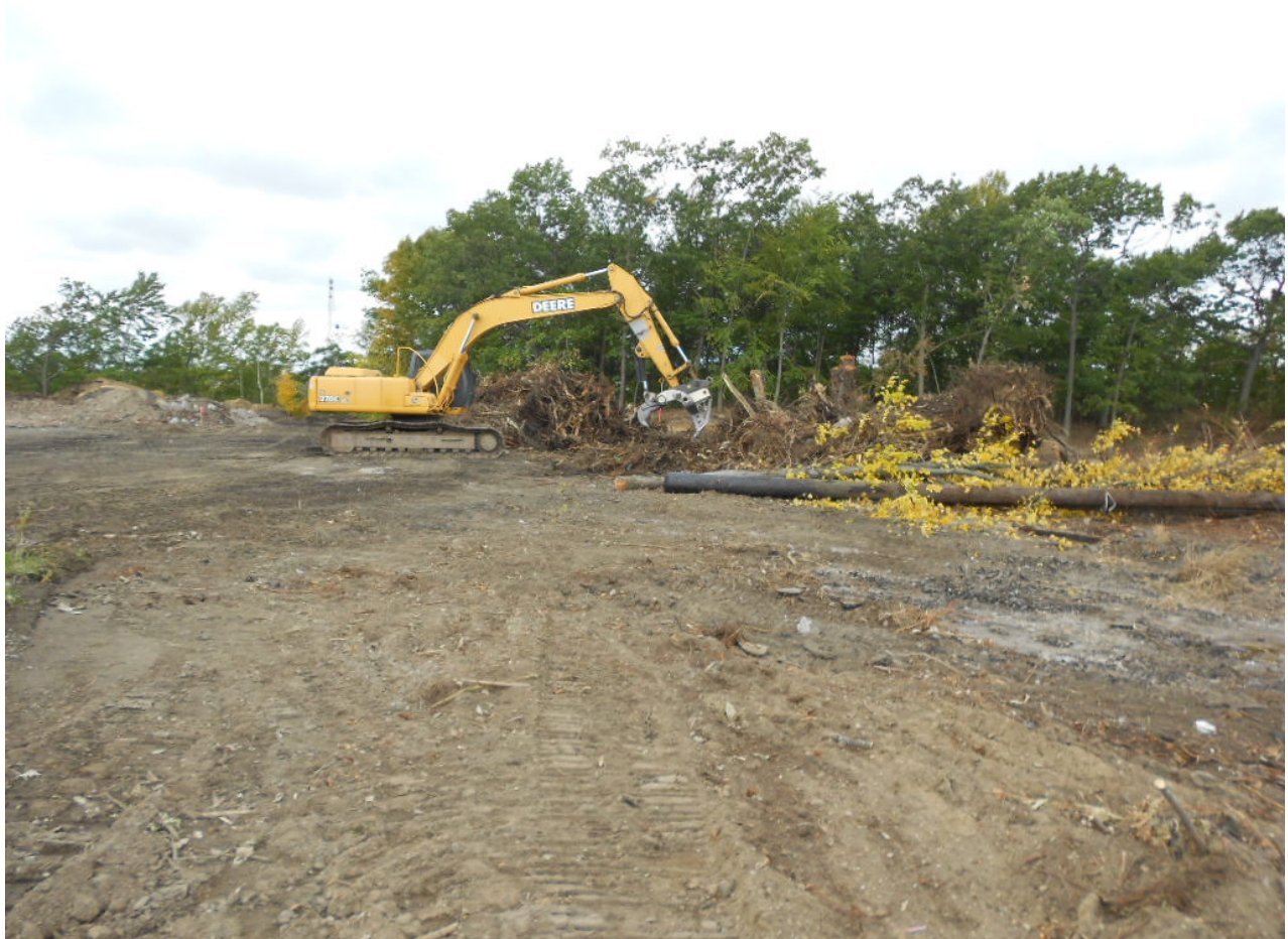
0953. Wagner Wood shearing stumps for chipping, looking west
