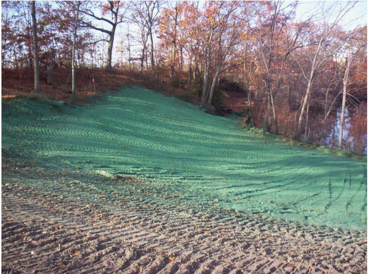
1665. Western side of Area 3 hydroseeded, looking northwest
