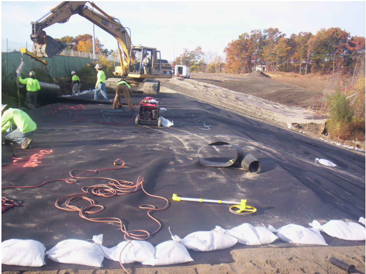
1581. Looking southwest at geomembrane installation at Area 4. Begin welding seams.
