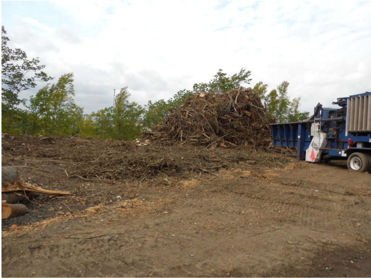
0950. Wagner Wood stockpiled sheared stumps for chipping
