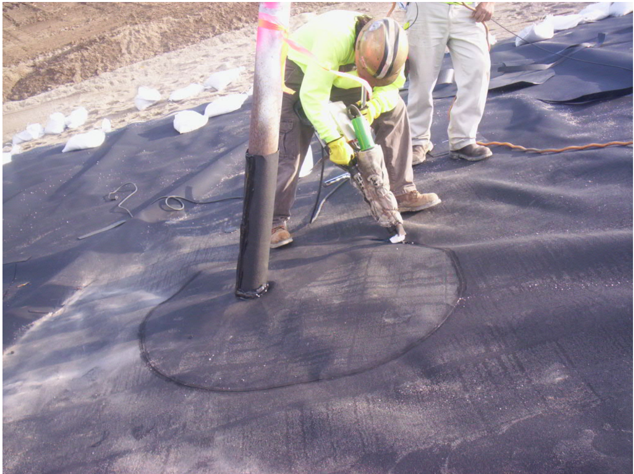
1586. Extrusion welding boot for monitoring well
