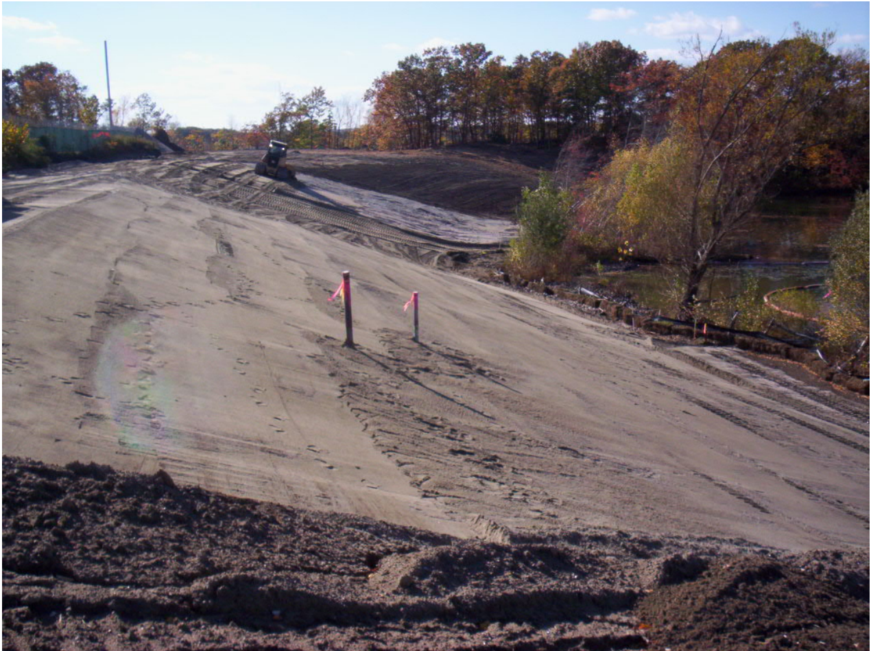
1575. Dozer repairing buffer sand at Area 4, looking southwest
