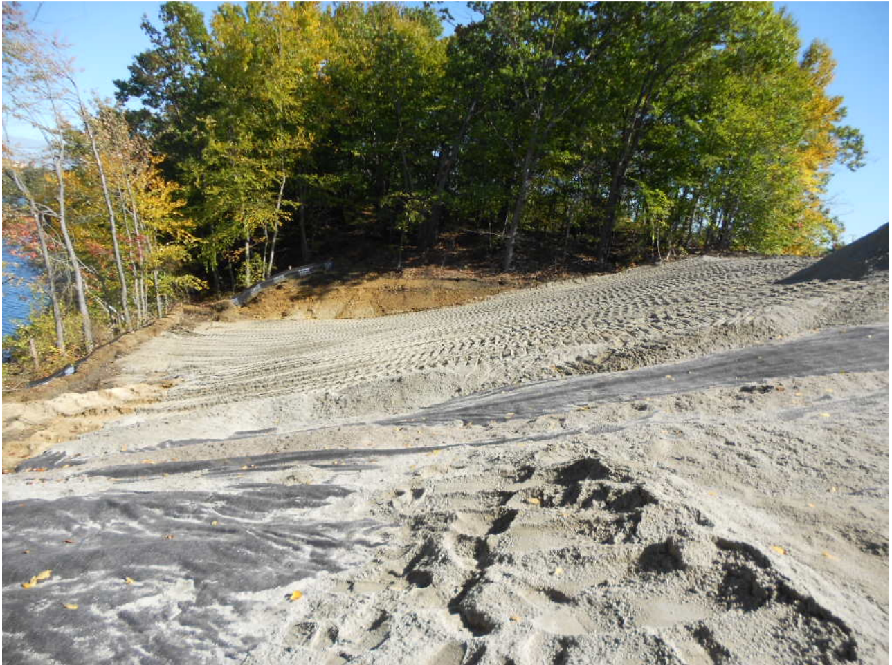
0968. Backfilling Area 2 with cover soil, looking north
