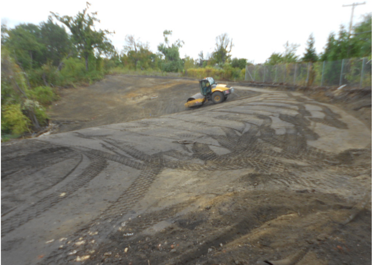
1029. Roller compacting sub-grade at Area 5, looking northeast
