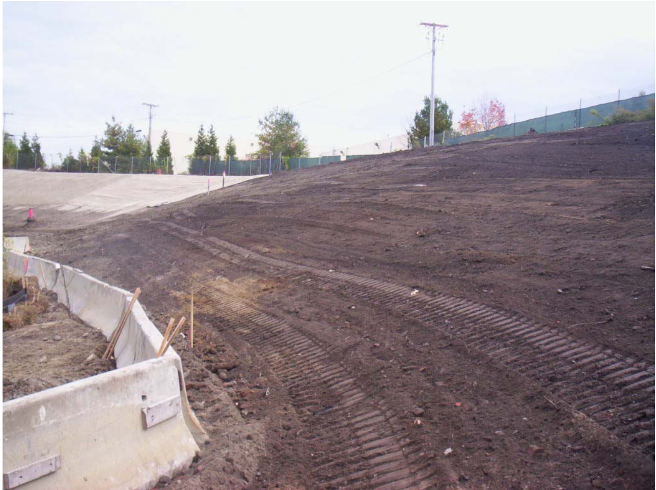
1051. Sub-grading achieved at Area 4, looking east
