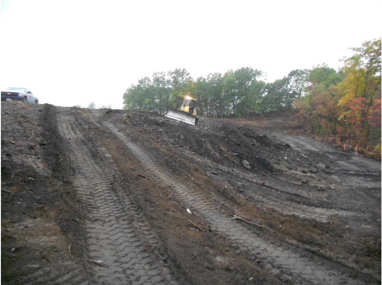
0994. Grading Area 3, looking southwest
