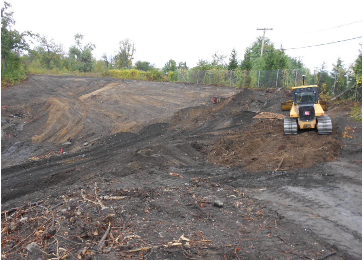
0967. Dozer grading sub-grade at Area 5, looking northeast
