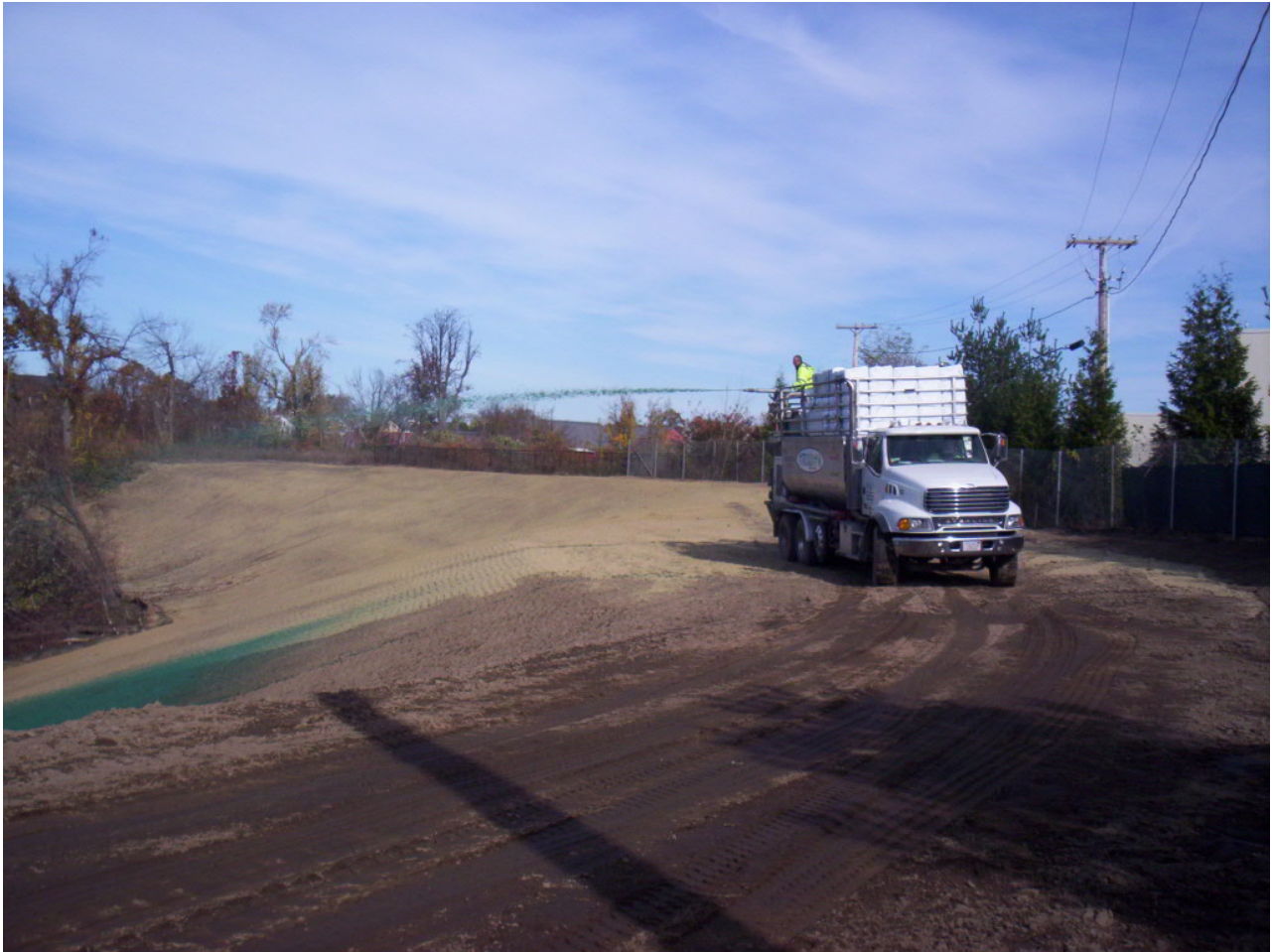
1662. Hydrograss hydroseeding Area 4, looking northeast
