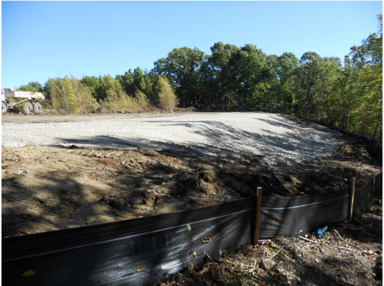
0977. Area 1 backfilled with cover soil, looking southeast
