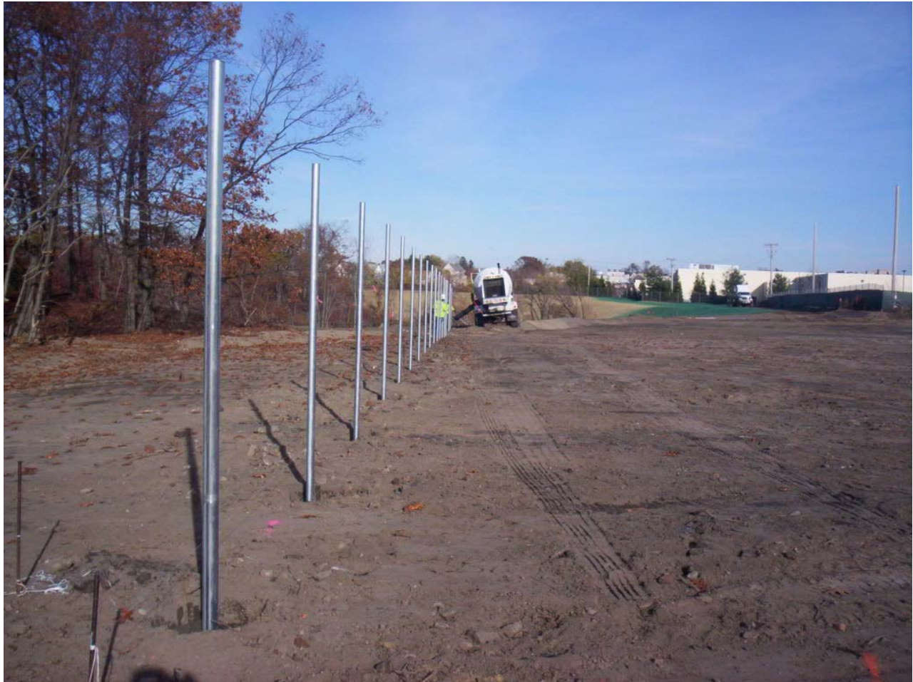
1668. Line of fence posts installed between Areas 2 and 3, looking northeast
