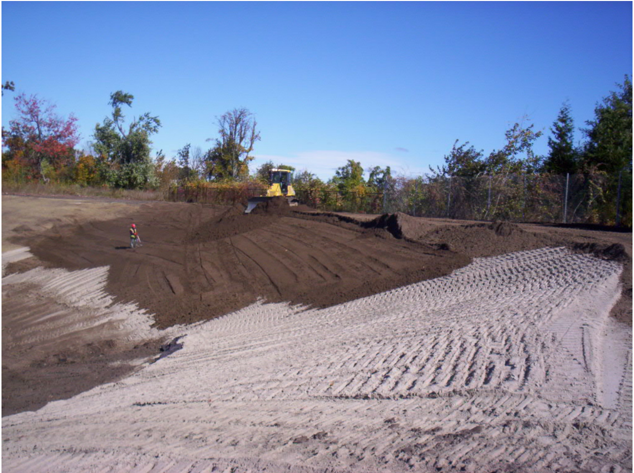
1554. Installing topsoil at the upland soil cap at Area 5, looking east
