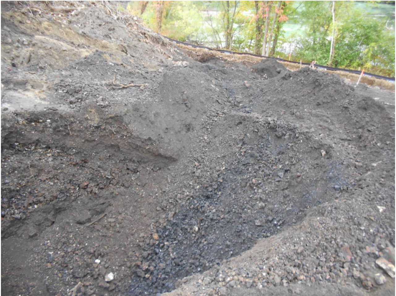
1006. Test pits in industrial fill area with volcanic rock looking material
