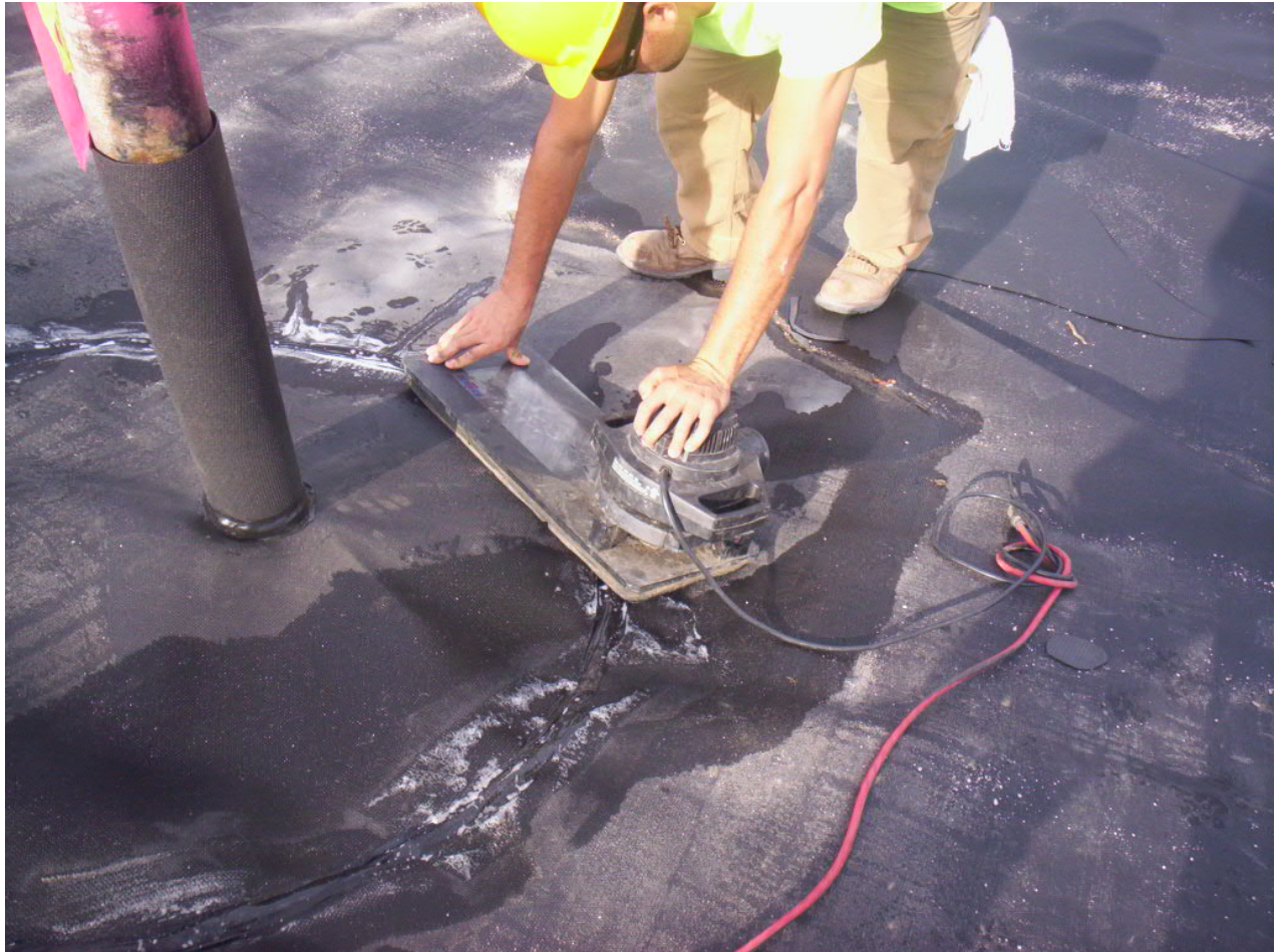
1593. Vacuum test for extrusion weld for boot at monitoring well
