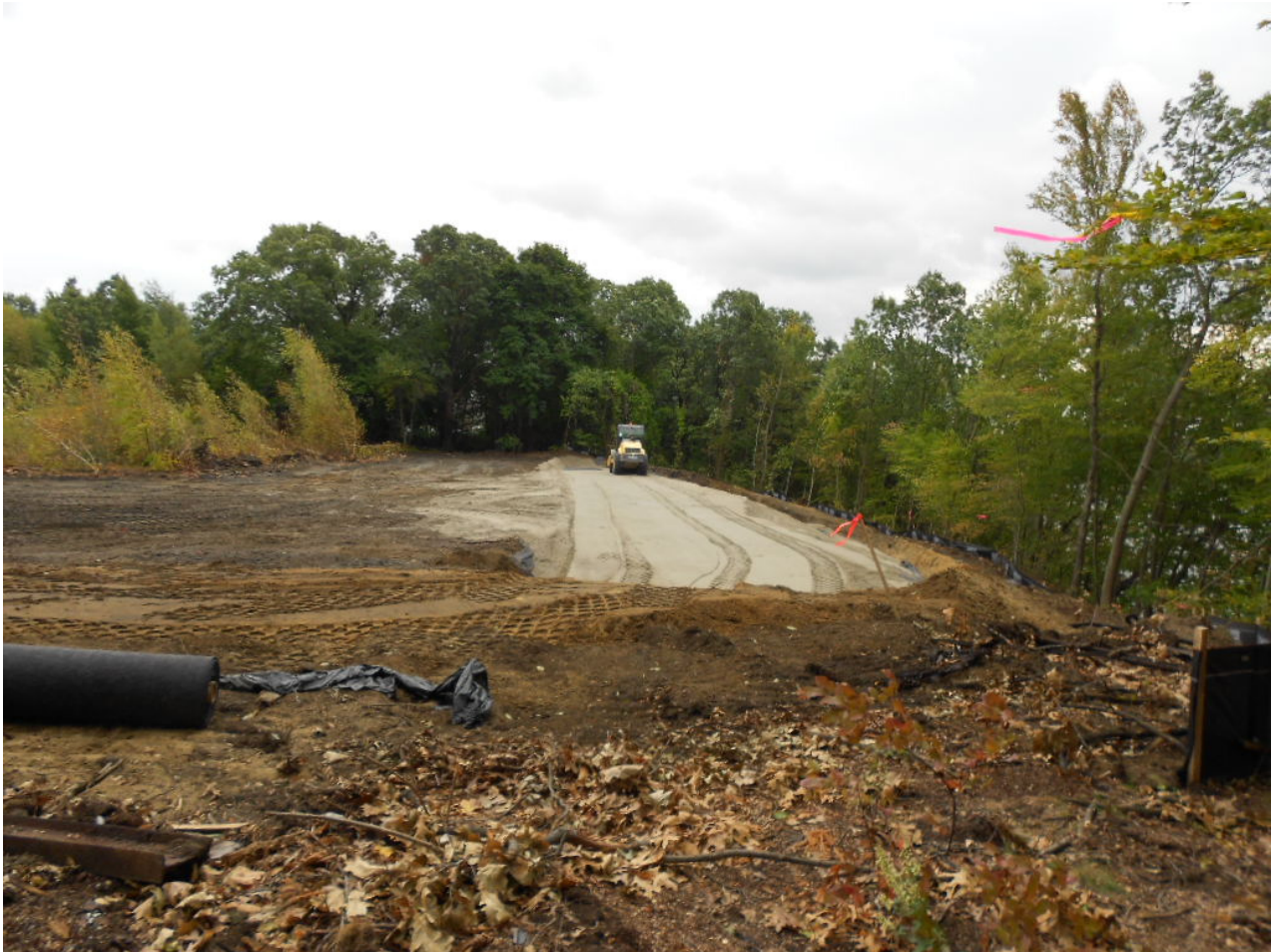
0954. Roller compacting cover soil at Area 1, looking south
