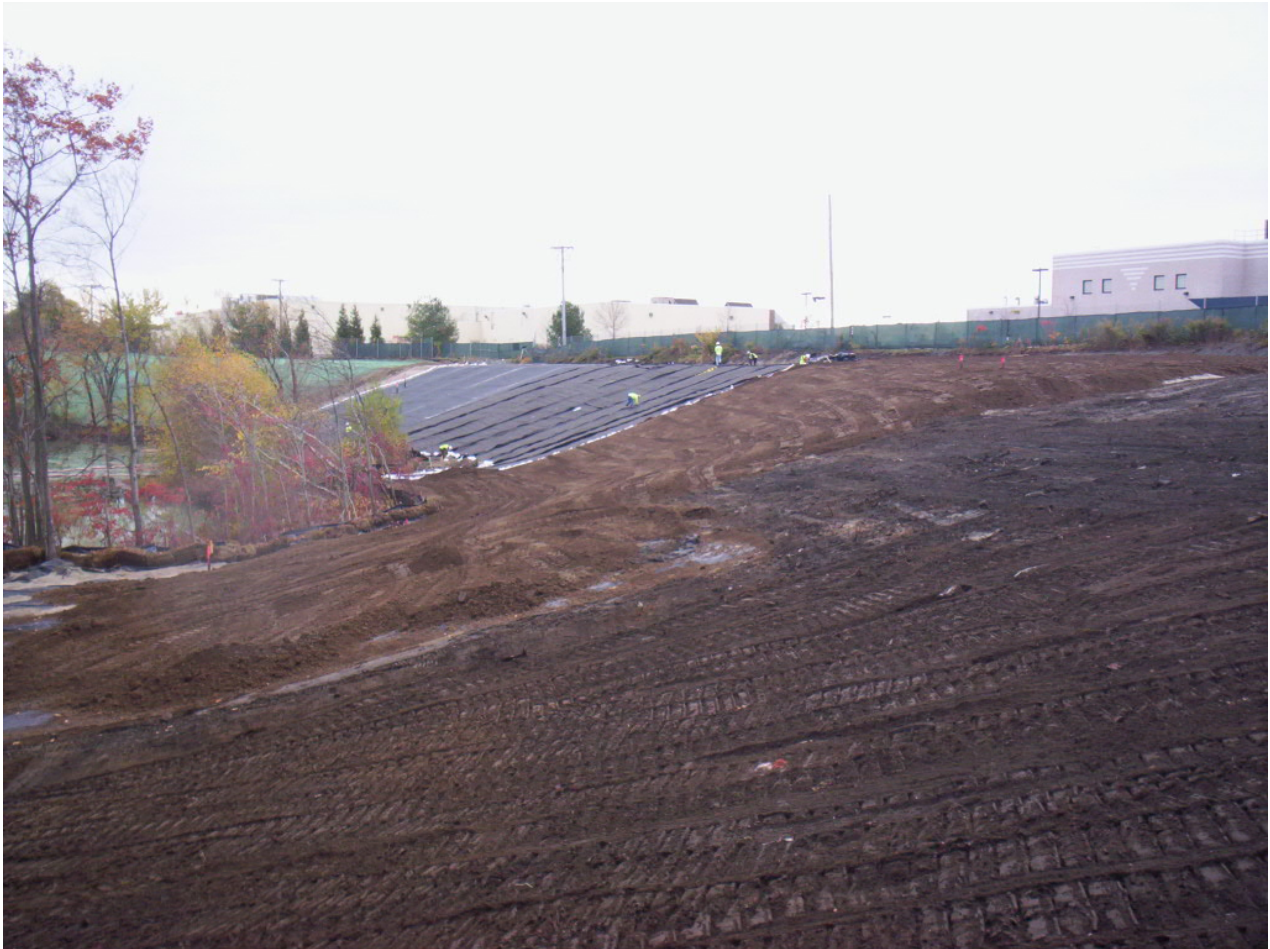
1607. Looking east at geocomposite installation at Area 4
