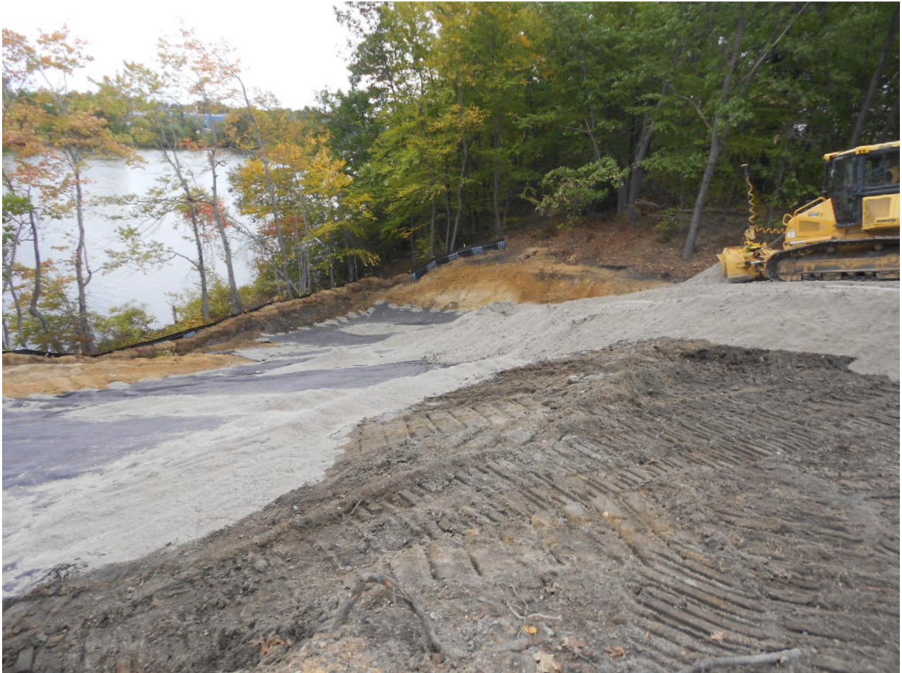
0965. Placing cover soil at Area 2, looking west
