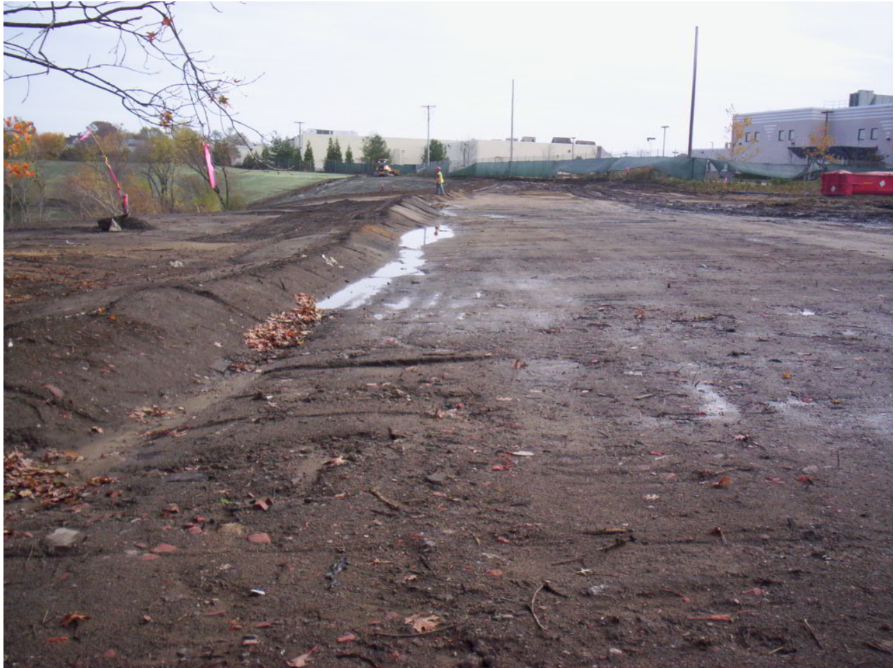
1625. The site was saturated the day after the hurricane, looking east
