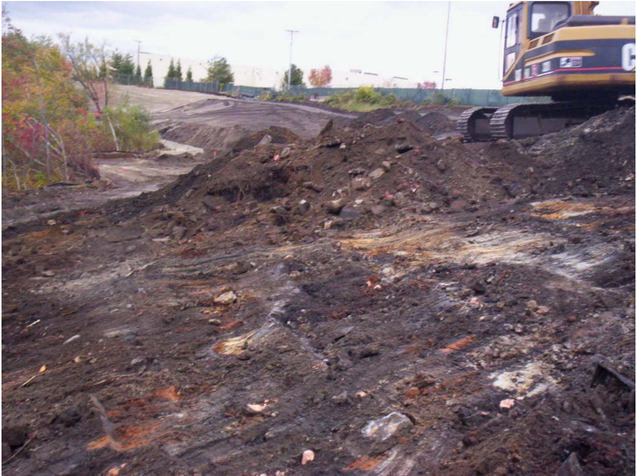
1044. Grading industrial debris with the excavator at Area 3, looking east
