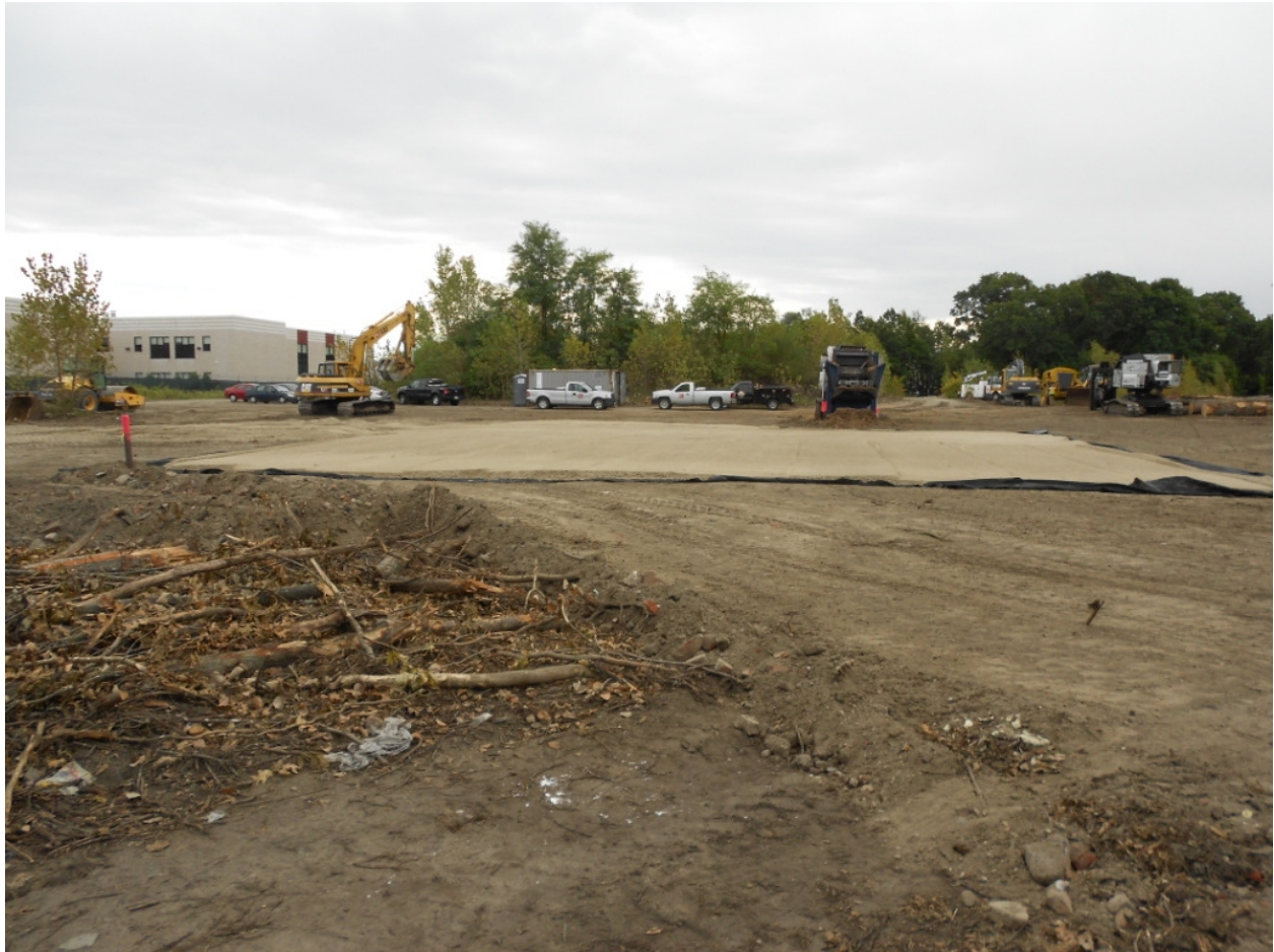
0921. Looking southeast at the lay down area
