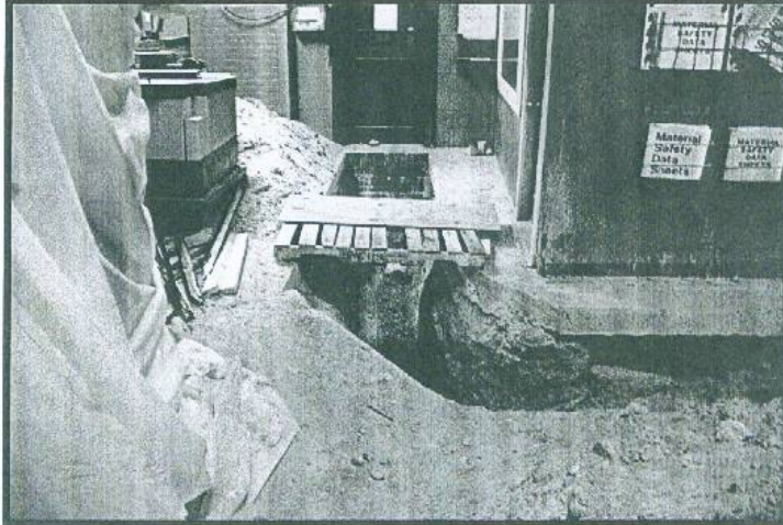
Photo No. 3 - New Sewer Main Trench approaching Basement under Dye Laboratory.
