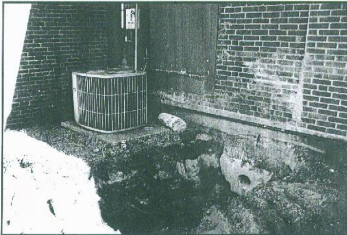
Photo No. 4 - New Sewer Main Location in rear Maintenance Area.
