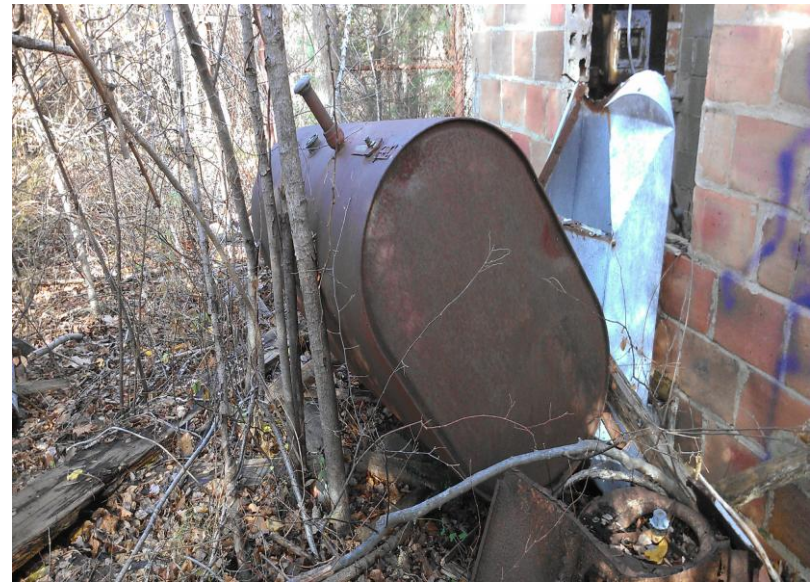
6) View of an abandoned AST located on the northeastern portion of the Subject Property.
