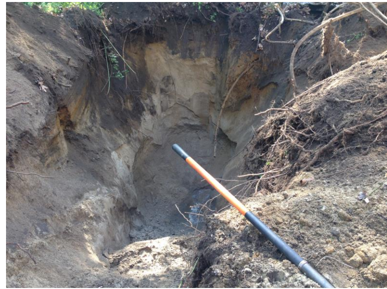
18) AOC-10: Coating Room. View of test pitting activities in AOC-10.
