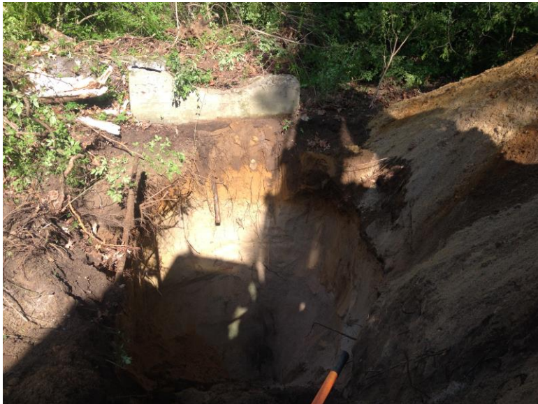
19) AOC-11: Acetone Tank. View of test pitting activities in AOC-11.
