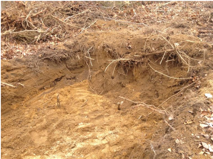
3) AOC-2: RCA-1 Excavation.
