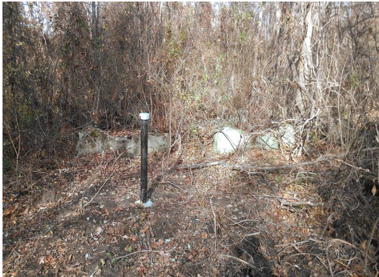
15) AOC-9: Solvent Storage Tanks. View of concrete tank cradles in AOC-9.
