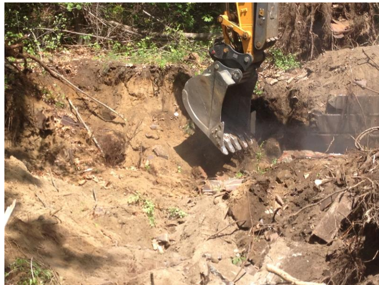
10) AOC-6: Drum Storage Area/Benzol House. View of AOC-6 excavation in progress.
