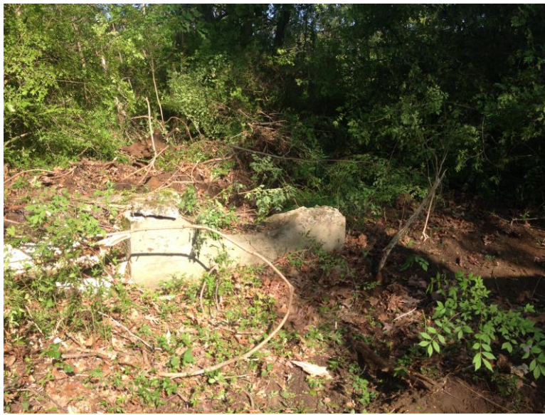
17) AOC-10: Coating Room. View of concrete tank cradles in the vicinity of the Coating Room.
