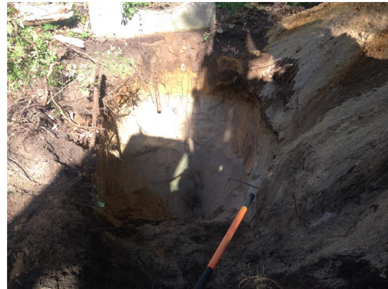
20) AOC-11: Acetone Tank. View of test pitting activities in AOC-11.
