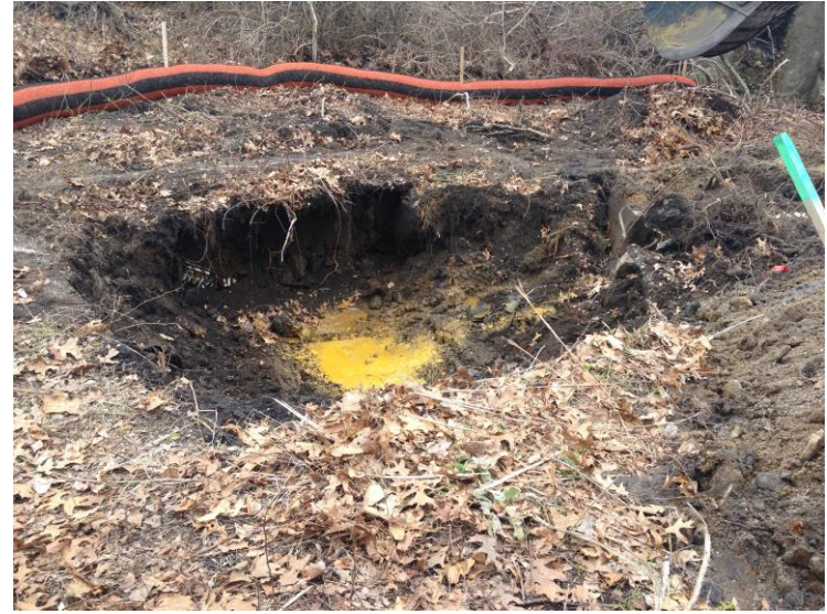
2) AOC-1: UST Area. View of final extent of UST excavation.
