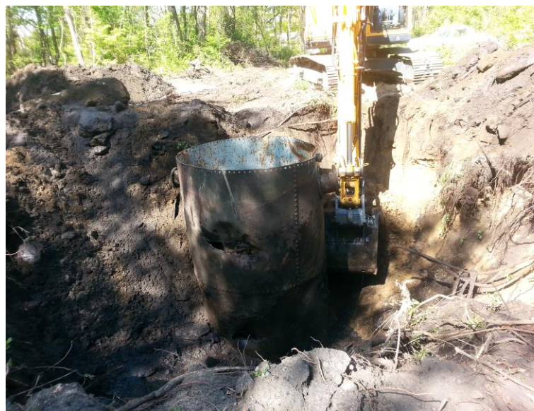
8) AOC-5: Cistern. View of Cistern excavation in progress.
