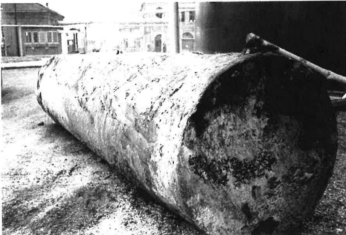
Excavated Tank #1 in good condition.
