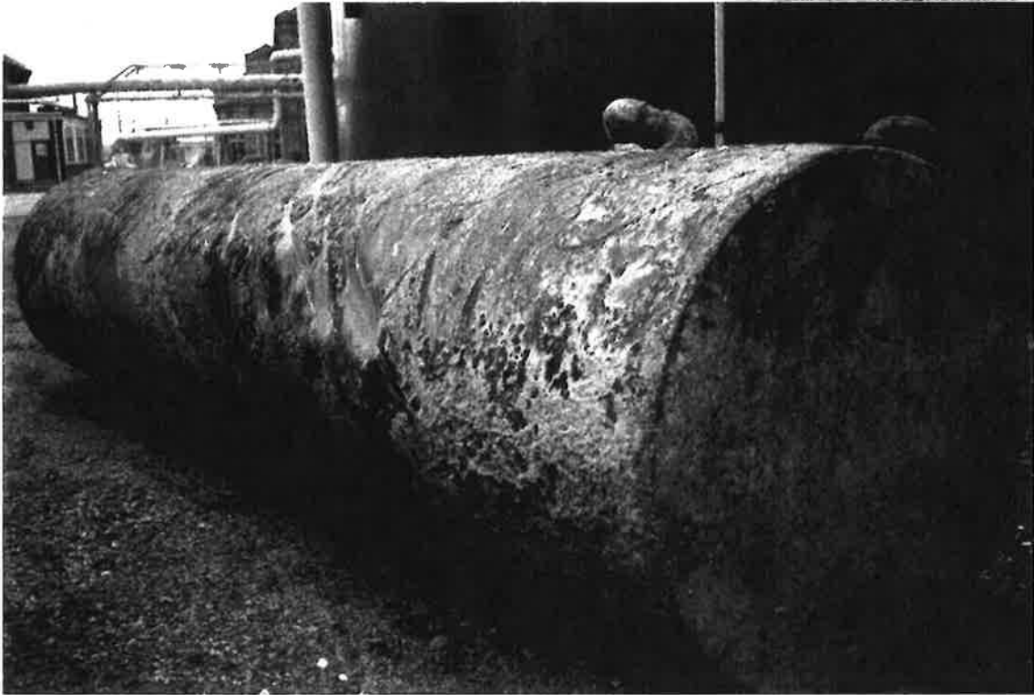
Excavated Tank #2 in good condition.
